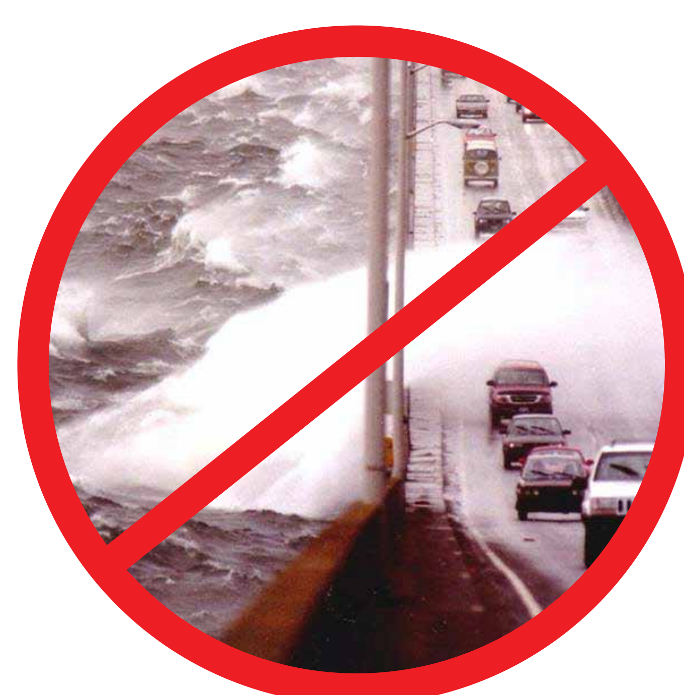
With a higher roadway, the new bridge won't provide free car washes during storms.
