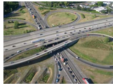
I-405 and SR 167 interchange, looking south
