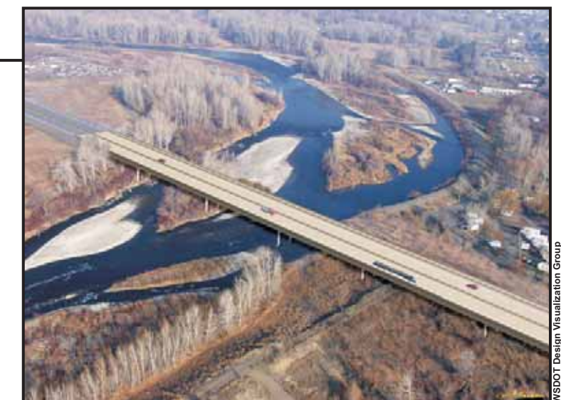
SR 24/Yakima River Bridge
