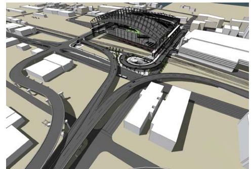
The project will provide a new off-ramp from I-90 to South Atlantic Street (the middle ramp in the west-facing simulation above) and an elevated crossing over the railroad tracks, with a loop ramp at Third Avenue South and South Royal Brougham Way. It will also make improvements to South Atlantic Street and its intersection with First Avenue South.
