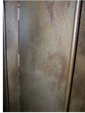
Day Tank Bulkhead, Frame-2 (D004.jpg)
