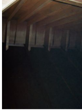
Storage Tank Overhead, Rub-rail and Bottom, Outboard At Top (S011.jpg)
