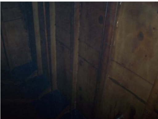
Storage Tank, Inboard, Bottom (S006.jpg)
