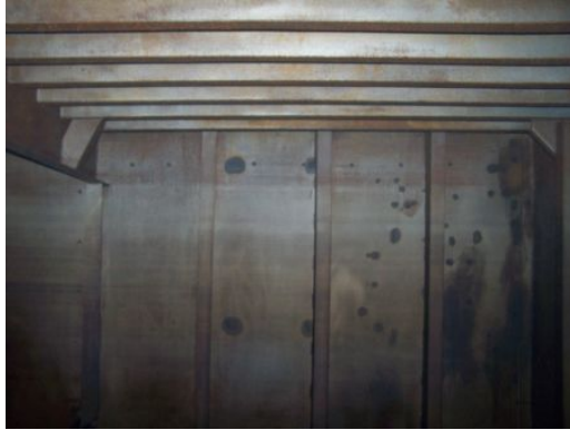
Storage Tank Bulkhead, #2 End Frame-6, Top (S003.jpg)
