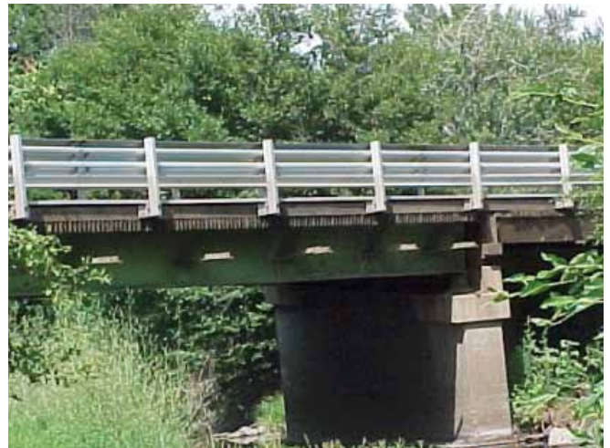
Side view of existing Satus Creek Bridge
