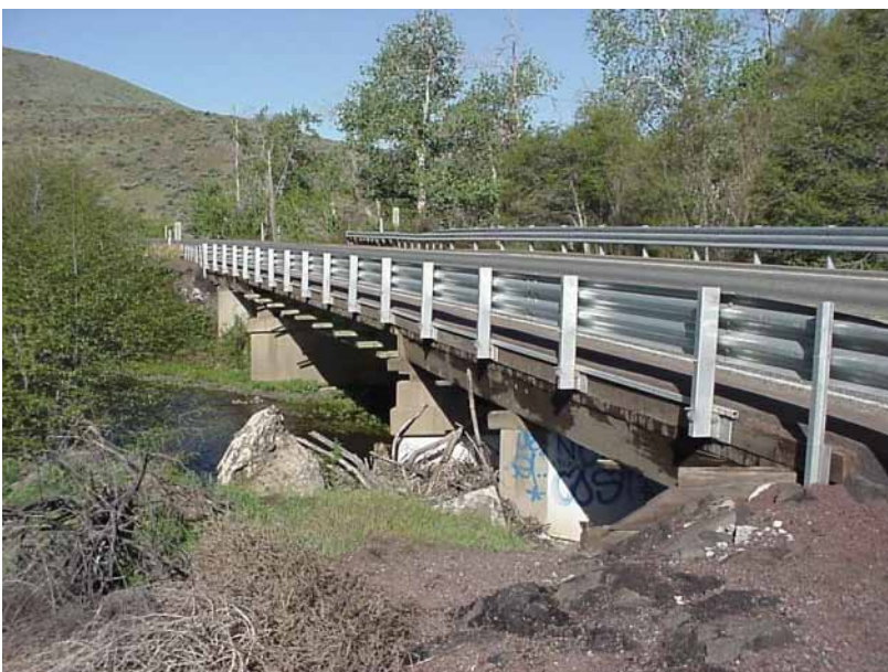
Existing Satus Creek bridge looking west
