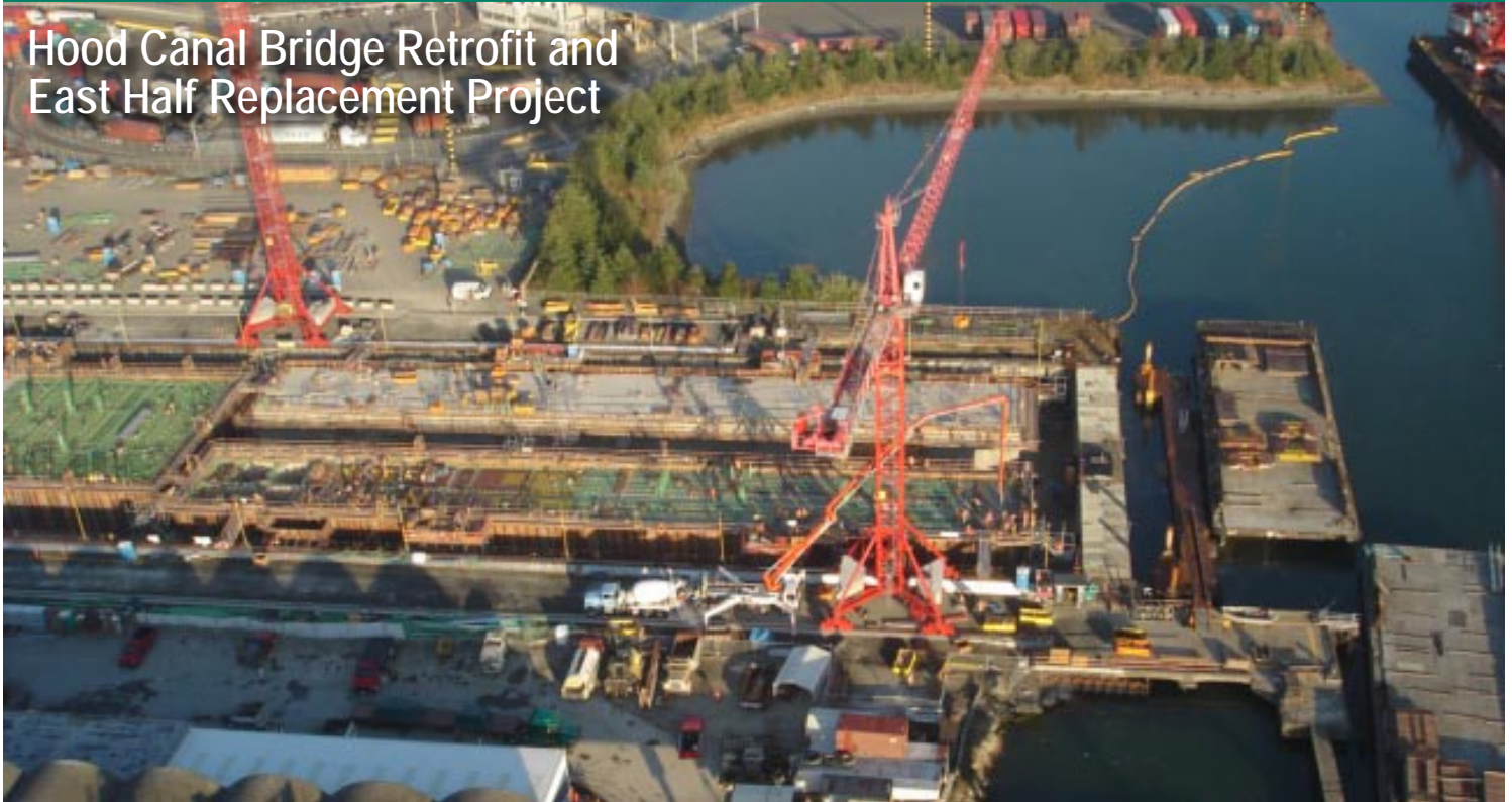
Crews pour concrete for the top deck of pontoon PB, September 27, 2006.
