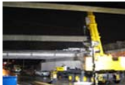
Crews place a girder for the Oakesdale bridge.
