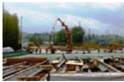
Crews place concrete for the new Oakesdale bridge
