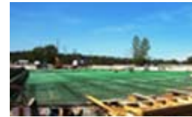
Crews tie rebar for the Oakesdale bridge deck.
