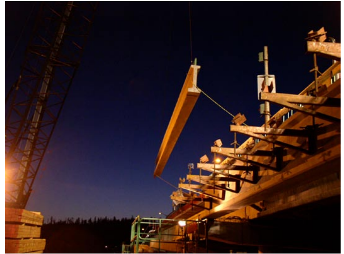
A crane places a girder for widening the west half. June 2004
