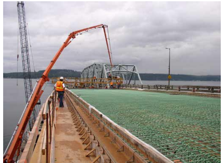
Crews place concrete for new west-half deck section. July 2005
