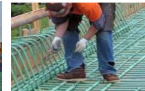
An iron worker ties rebar for the Oakesdale bridge
