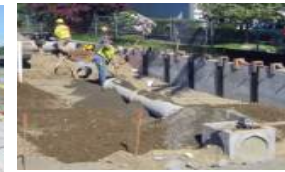
Crews install drainage structures along southbound I-405.
