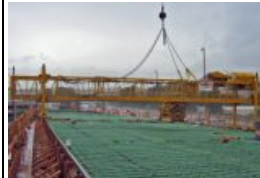
A BidWell paving machine waiting for concrete.
