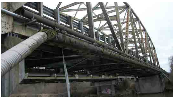
Both spans of the Interstate 5 Nooksack River Bridge near Ferndale (pictured above) are scheduled for painting in 2014. To protect the bridge for years to come, crews will remove rust, old paint and other debris, and put on fresh coats of primer and paint.
