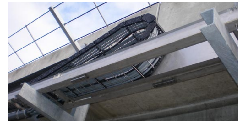
The west-half cable track is in place, October 26, 2007.
