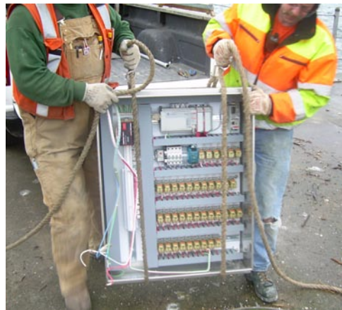
Workers move an interface panel into place.
