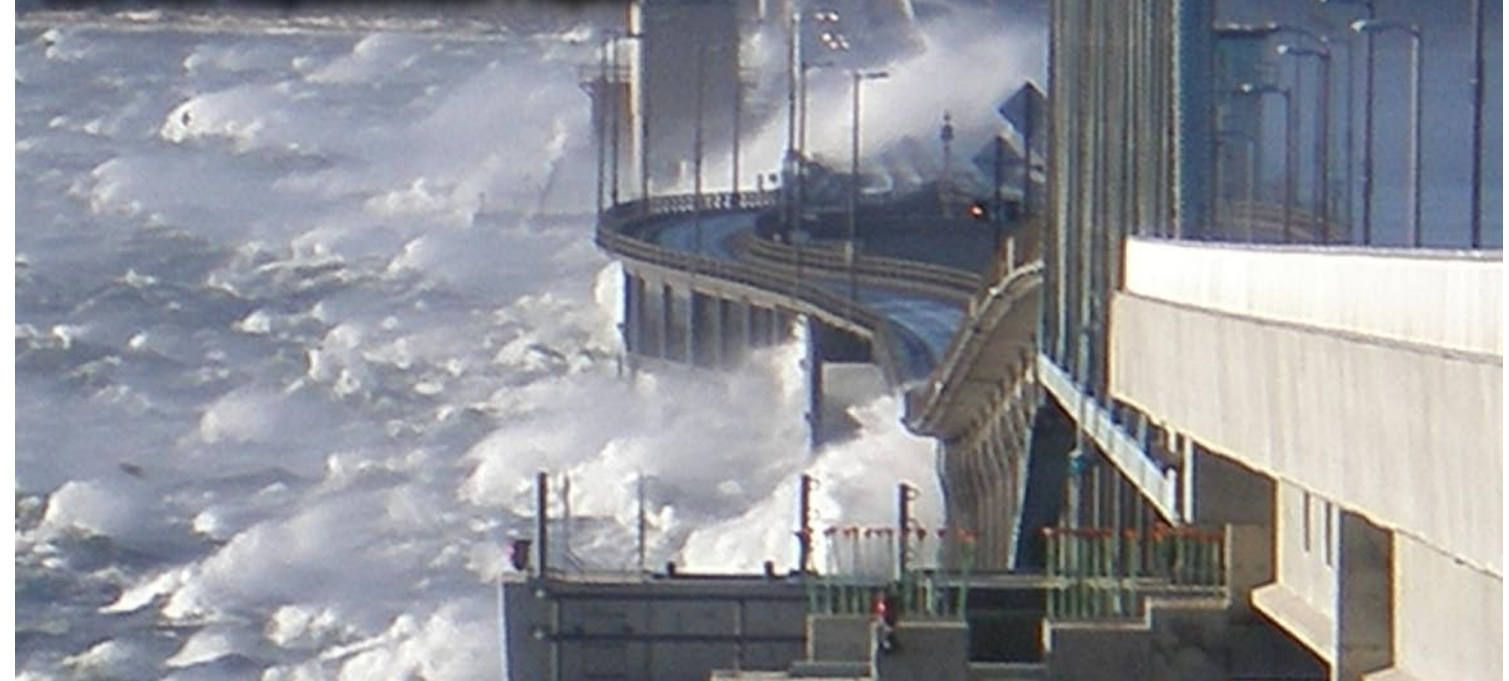
Hood Canal Bridge weathers winter storm, October 18, 2007.
