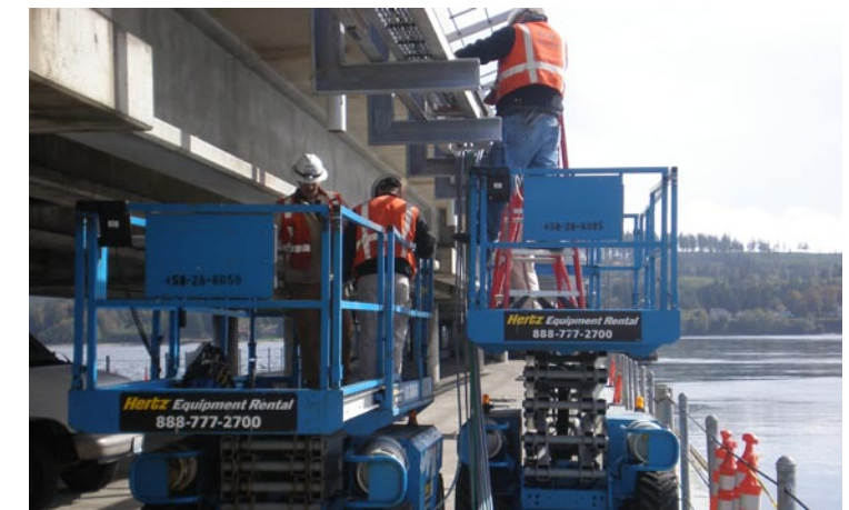
Electricians install the electrical cable in the track, October 8, 2007.
