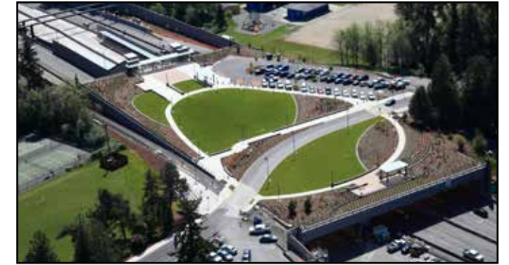
The Evergreen Point Road lid includes a median transit stop (upper left), one of two on the Eastside corridor.
