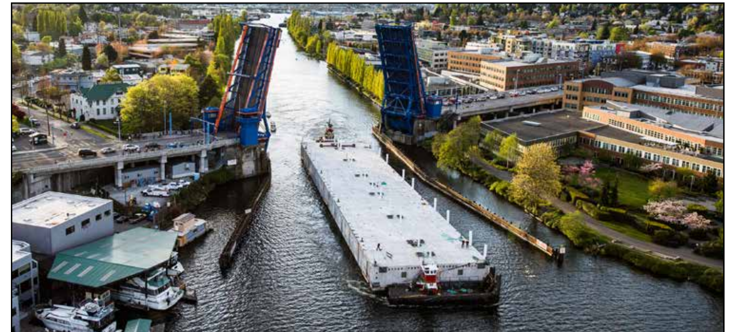
Pontoon F, the final pontoon needed for the new floating bridge, travels through the Seattle ship canal in April 2015 en route to Lake Washington. The new floating bridge opened to traffic in April 2016.
