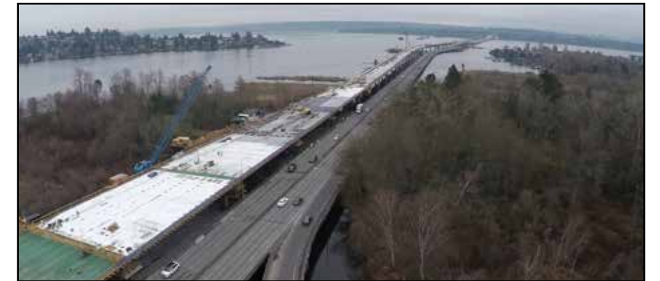
February 2017 view of West Approach Bridge North construction across Union Bay.
