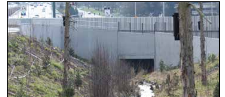
New culverts built under SR 520 are designed to aid fish migration.
