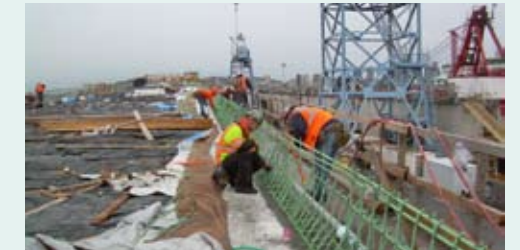
Ironworkers place span rebar on pontoon UWX. Feb. 10, 2009.
