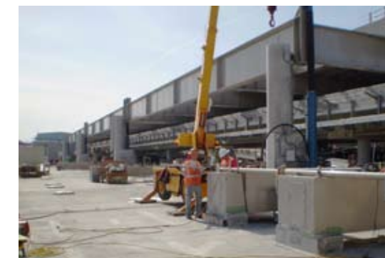
The lift spans are elevated during tests. March 13, 2009.
