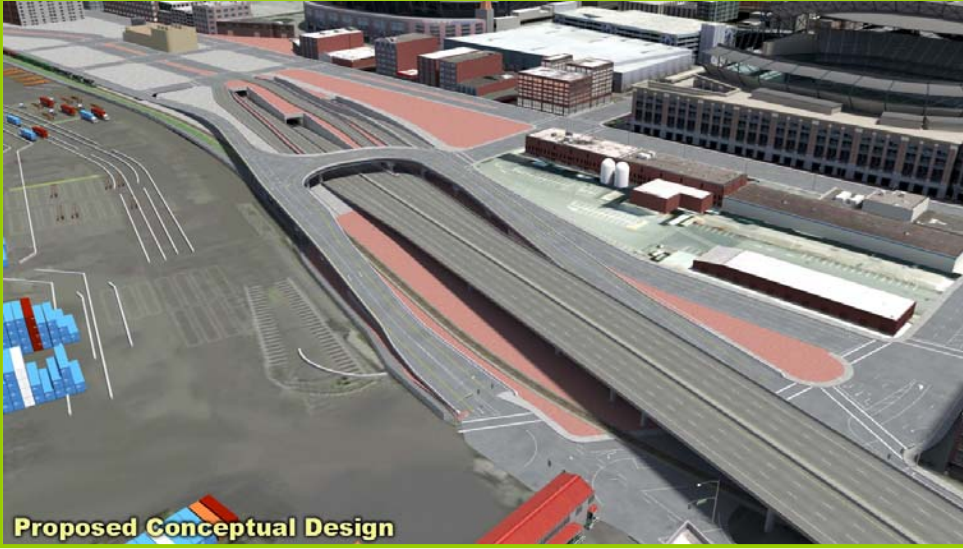
Looking northeast at proposed above-grade crossing and Alaskan Way S. to East Marginal Way S. connector, which ends prior to S. Atlantic Street.
