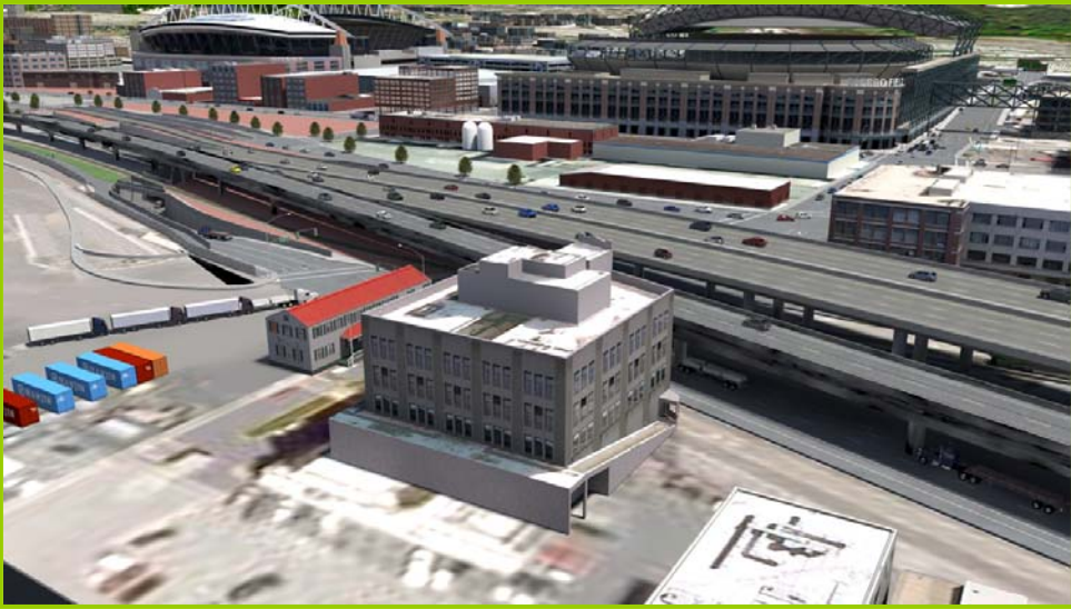
Looking east at Alaskan Way S. to East Marginal Way S. connector, which extends past S. Atlantic Street (not shown in left graphic).
