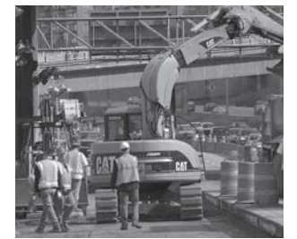
I-5 Pavement Rehabilitation Project in Seattle, completed in 2005.
