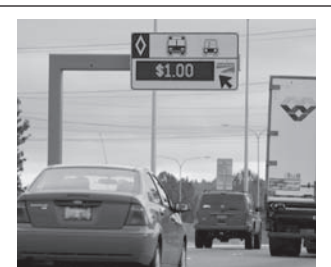
SR 167 HOT lanes pilot project opened to traffic spring 2008.
