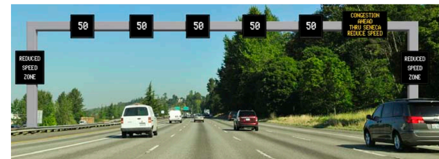
Speed limit signs automatically reduce speed and warn drivers of backups ahead.
