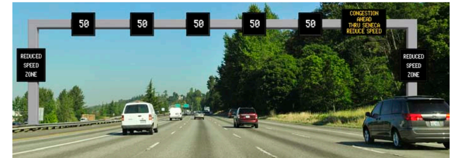
Speed limit signs automatically reduce speed and warn drivers of backups ahead.
