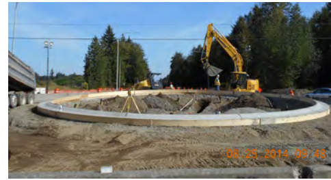
The new roundabout at 84th Street NE under construction in August 2014.
