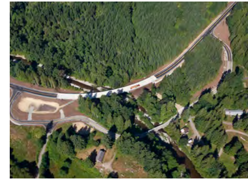
The new Pilchuck River Bridge opened to traffic in May 2014.
