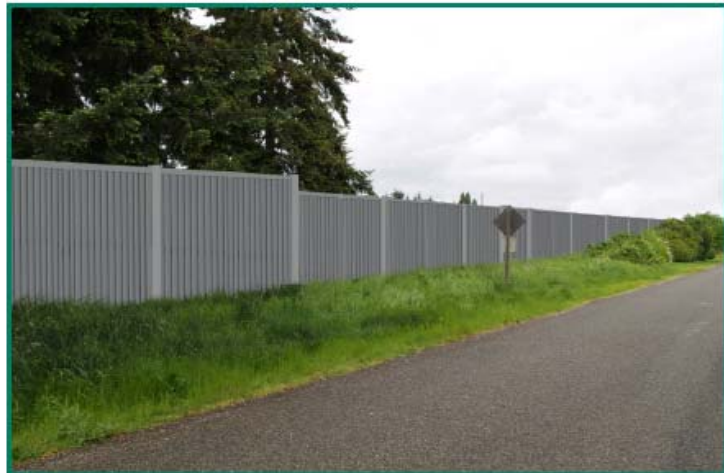
Preliminary design concept showing Carsonite AcoustaShield. View of 1st Avenue NE looking north.
