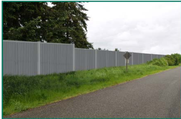
Preliminary design concept showing Carsonite AcoustaShield. View of 1st Avenue NE looking north.
