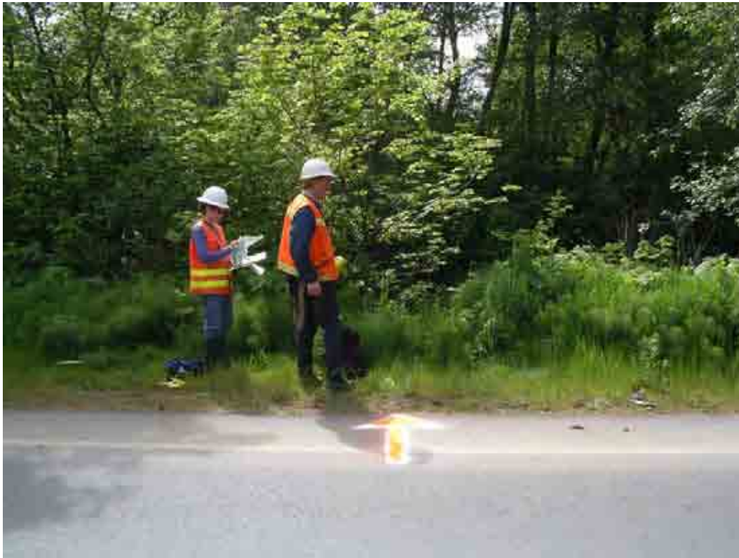
Photo A-68. Pysht River Site ID P-7 Bank erosion (right bank) 42 year extent. 13 feet to edge of pavement. (Photo 2422)
