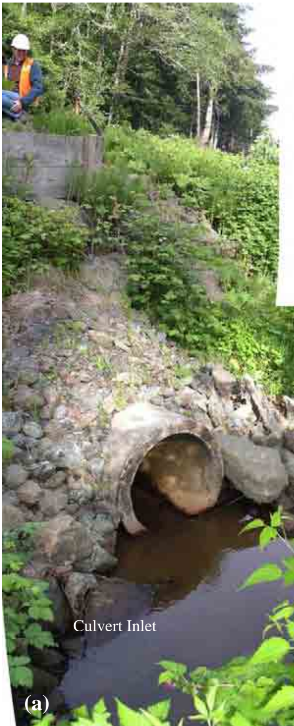
Photo A-11. Hoko River Site ID H-2 (May 12, 2005) (a) Upstream side of undersized culvert. (b) downstream side of culvert. Culvert is 24 inches in diameter. (Photo Pan 2528-2529 and Pan 2525-2526)
