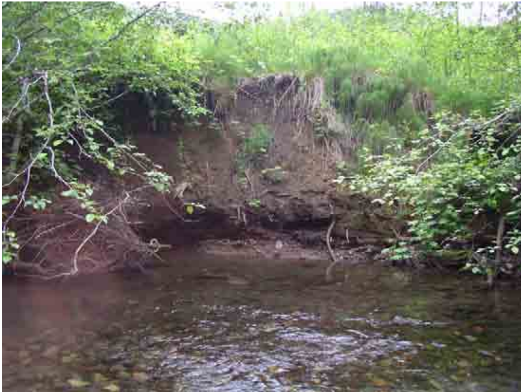
.Photo A-73 Bank erosion into fill material within the road prism of the historical alignment of State Route 112 at RM 5.9 on the Clallam River (May 11, 2005). The bank height is 10 feet and the banks consists of sand and gravel fill material over alluvial cobble, gravel and sand that typically makes up unmodified stream banks in the study reach. The flow direction is from right to left. (Photo-2368)
