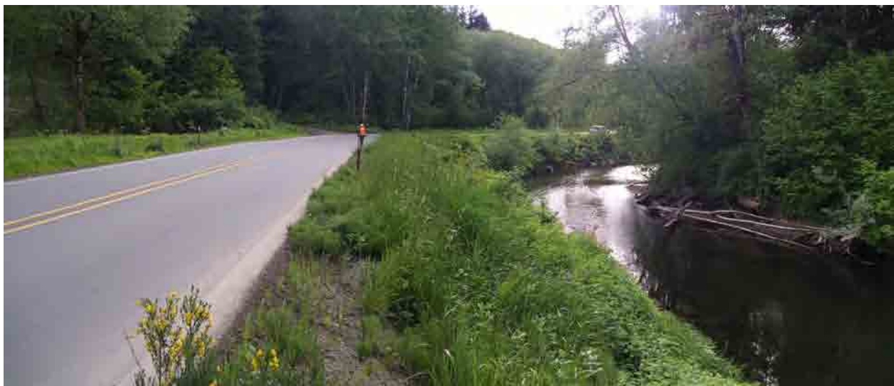
Photo A-46. Pysht River Site ID P-4 (May 11, 2005). Looking downstream on the Pysht River at milepost 28. (Photo 2449-2450)
