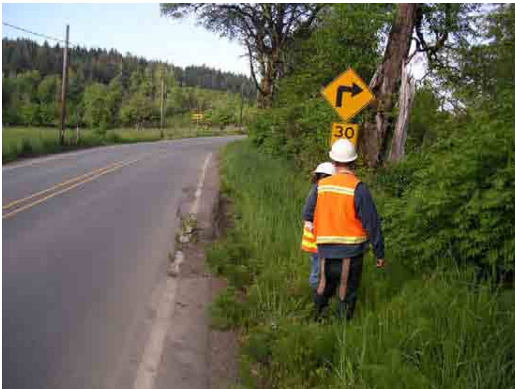
Photo A-30. Pysht River Site ID P-3 (May 11, 2005). Looking downstream. Bank erosion, cracked pavement, top of bank is 10 feet from the edge of pavement. (Photo 2499)
