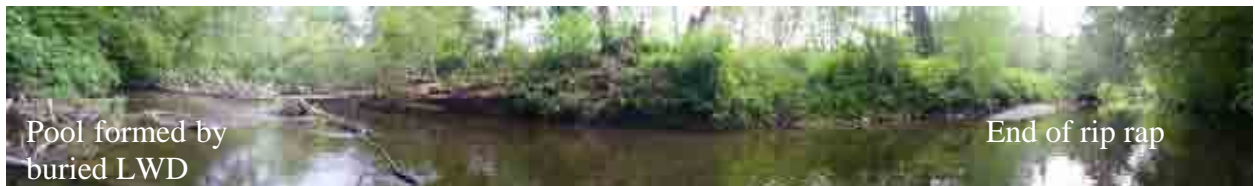
Photo A-43. Pysht River Site ID P-4 (May 10, 2005). Just downstream of MP 27. downstream of rip rap is an unprotected bank ~18 feet high. (Photo Pan 2437-2443)
