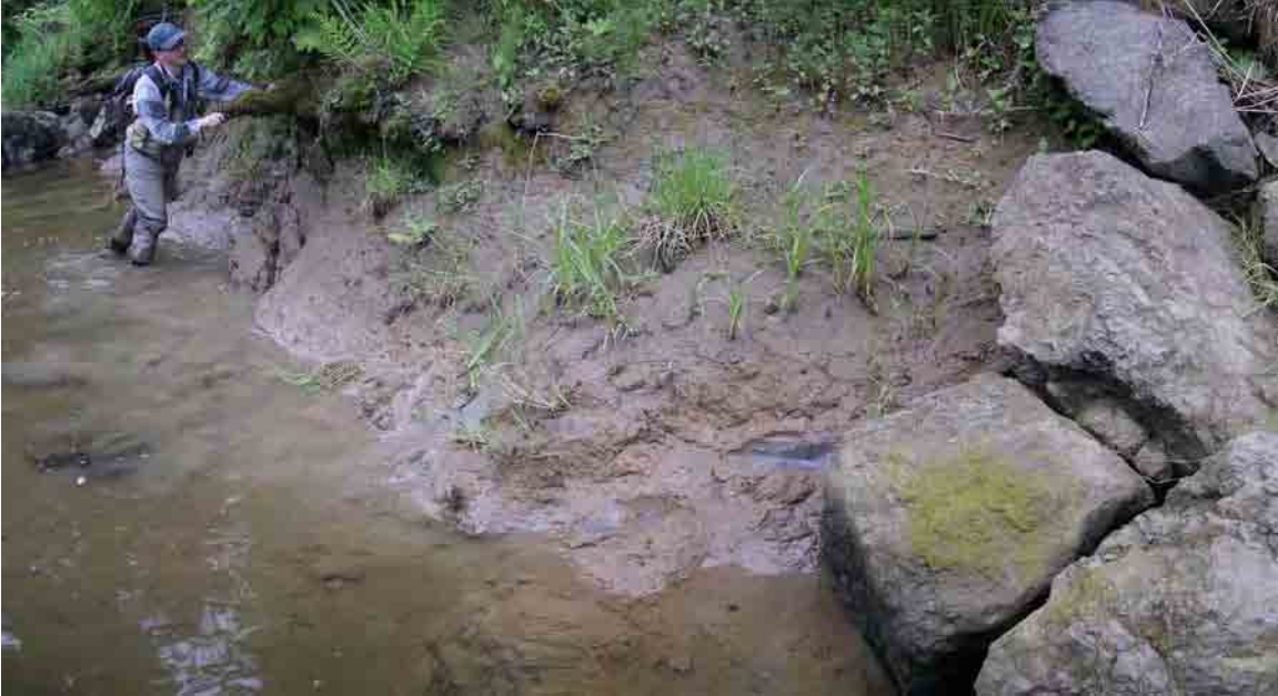
Photo A-72. Site ID P-8. Taken at the toe of bank (~6ft from edge of water on rock). (Photo 2275-77)
