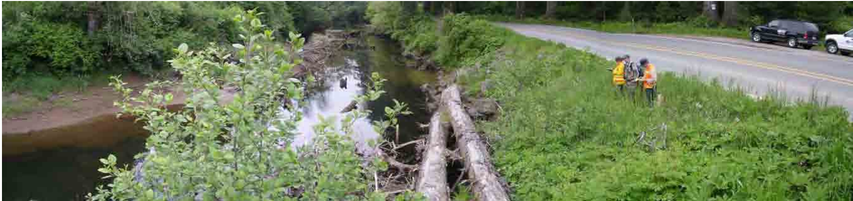
Photo A-70 Pysht River Site ID P-8 (May 10, 2005). Bank erosion (RB), rip rap at site (some falling), 75-foot rip rap launching, 27-feet of bank slumping, and less than 10 feet EOP. TA notes: From sitka stump u/s end of site. Functional rip-rap is ~95 feet long about 40 feet beyond rip rap is at risk. (Photo Pan 2267-70)
