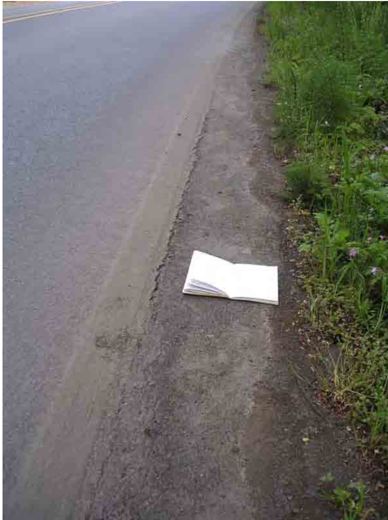
Photo A-26. Pysht River Site ID P-1 (May 12, 2005). Cracked pavement. (Photo 2778)
