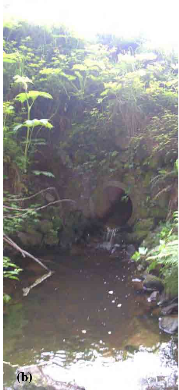
Photo A-11. Hoko River Site ID H-2 (May 12, 2005) (a) Upstream side of undersized culvert. (b) downstream side of culvert. Culvert is 24 inches in diameter. (Photo Pan 2528-2529 and Pan 2525-2526)
