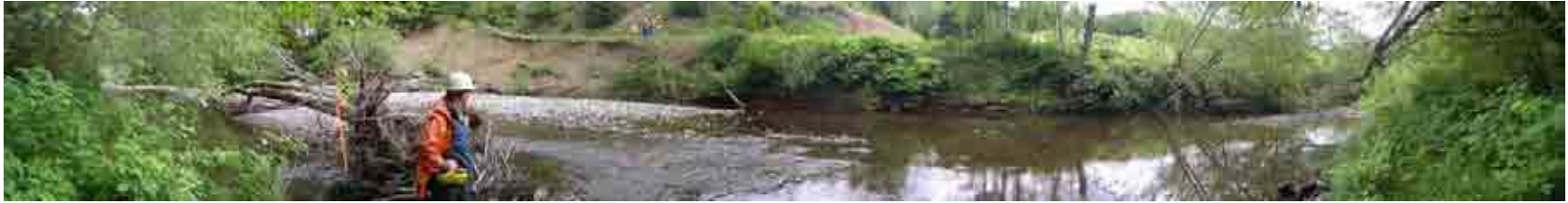
Photo A-16. Clallam River Site ID C-2 (May 11, 2005). Looking at the right bank. Erosion. Toe of slope erosion. (Photo Pan 2388-2394)
