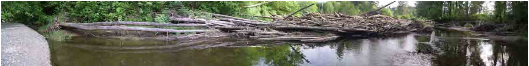
Photo A-53. Pysht River Site ID P-4 (May 11, 2005). Channel spanning logjam (Photo Pan 2487-2493)
