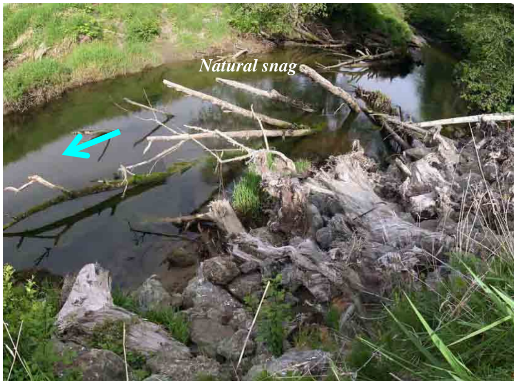
Figure A-4. Hoko River Site ID H-1 (May 12, 2005). Natural snag adjacent to bank protection work done in 2003(?) using rip and cabled stumps to stabilize left bank along SR 112. (Photo Pan 2541-2550)
