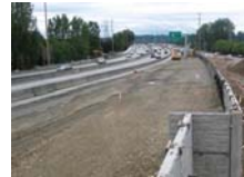
The sub grade to the west approach to the Oakesdale bridge
