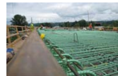
The rebar cage for deck for the new Oakesdale bridge
