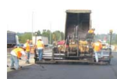
Crews placing HMA pavement
