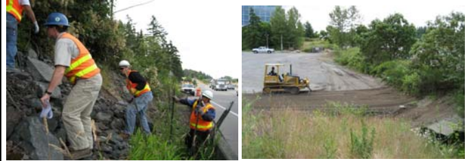
Establishing clearing limits prior to construction and preparing storage yard
