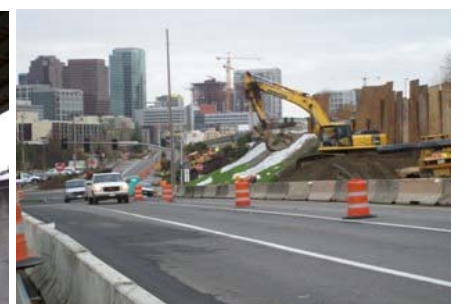
Dirt work at wall 2070, near SE 8th street
