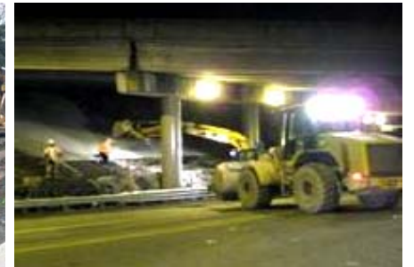
Constructing rock wall and slope protection at Coal Creek Parkway
