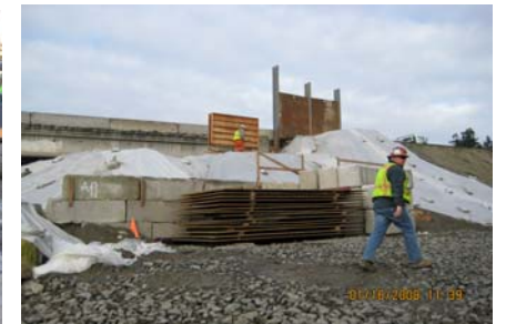
Crews demonstrate proper erosion control methods at Pier 3, CCP.
