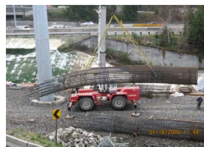
Crew member relocates rebar cage in preparation to set at Pier 5.
