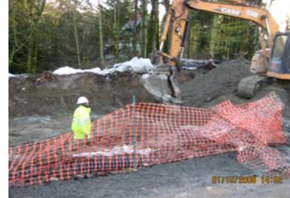
Construction of sediment pond at Wall 2105 to accommodate runoff.
