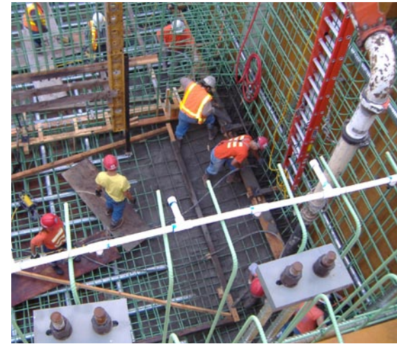
Workers pour pontoon PA floor concrete. May 19, 2006
