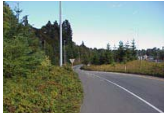
Figure 9-Henderson/City Center Ramp (looking back)
