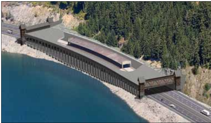
Reduce avalanche closure delays by building a new expanded snowshed. Visual concept comparison of the new and old snowshed.
