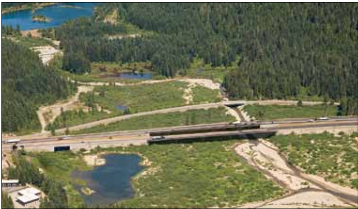
WSDOT will expand the bridges over Gold Creek for water and wildlife passage. Visual concept of the wildlife undercrossing and 1100'/900' bridges to be open to traffic 2013.
