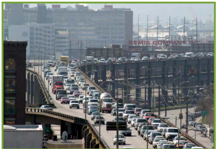
The Alaskan Way Viaduct has stood along Seattle's waterfront since the 1950s. The two-mile long structure is earthquake-damaged and must be replaced.
