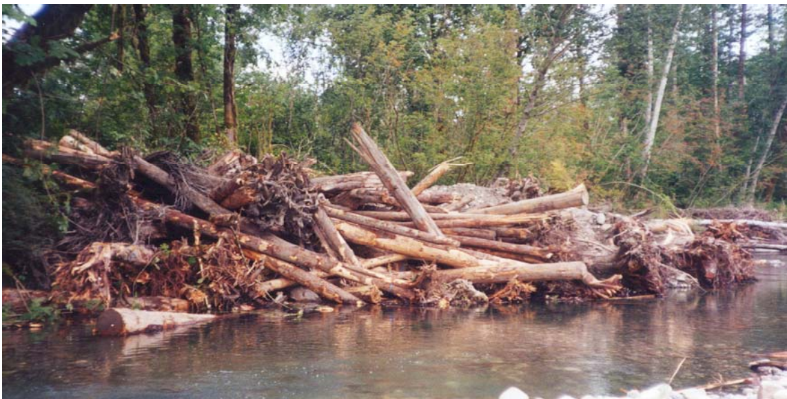
Figure I-7: ELJ constructed as part of the North Fork Stillaguamish, ELJ project.
