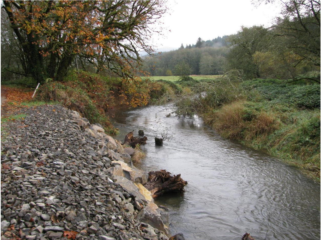
Figure 2. Bank repair on Nelson Creek, Wahkiakum County, looking north.
