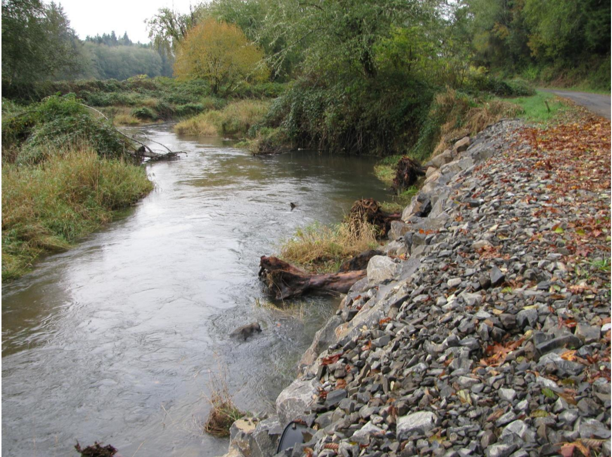
Figure 3. Bank repair on Nelson Creek, Wahkiakum County, looking south.
