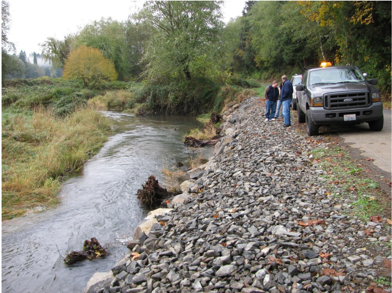
Figure 4. Bank repair on Nelson Creek, Wahkiakum County, people for scale.
