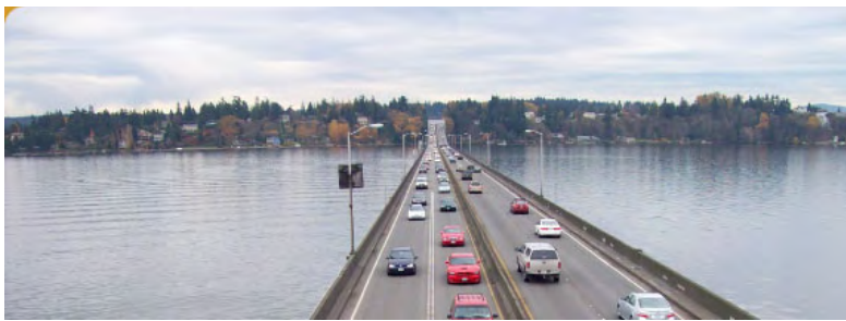
SR 520 Bridge—Existing Conditions
