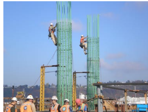
Ironworkers install column rebar on the new east-half draw span, Oct. 30, 2007.
