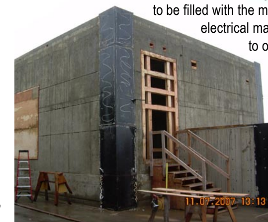
Crews remove forms from west-half electrical building, Nov. 7, 2007.
