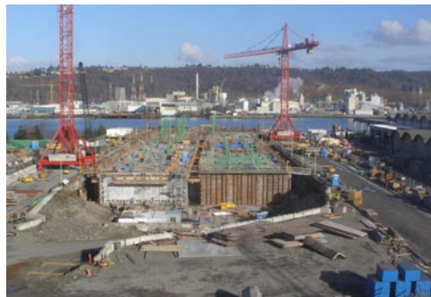
Four more Hood Canal Bridge pontoons are nearing completion, Dec. 31, 2007.
