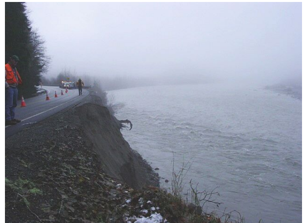
Figure 4. Streambank damage at SR 530 CED site (date of photos 11/19/2003).
