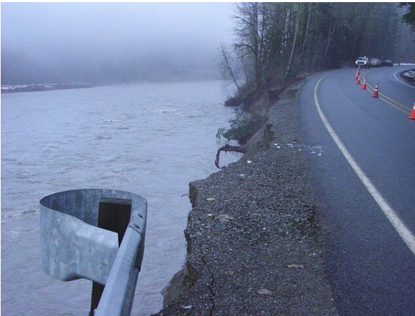
Figure 4. Streambank damage at SR 530 CED site (date of photos 11/19/2003).
