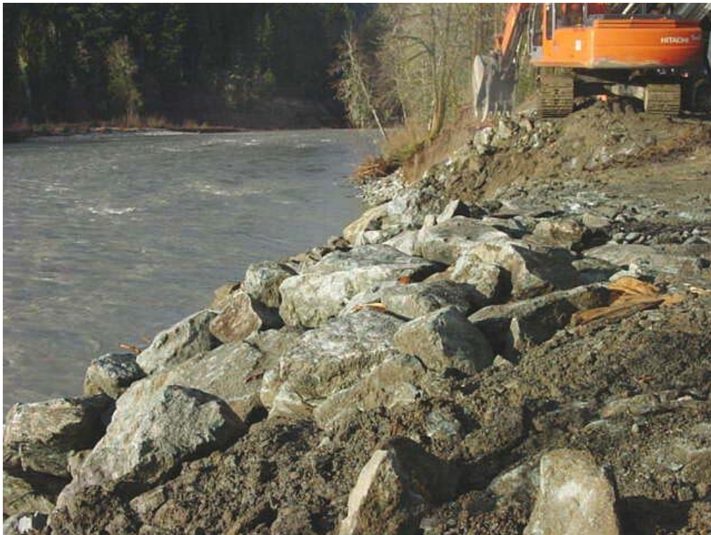
Figure 2. Installation of riprap at SR 530 CED site (November 2003).
