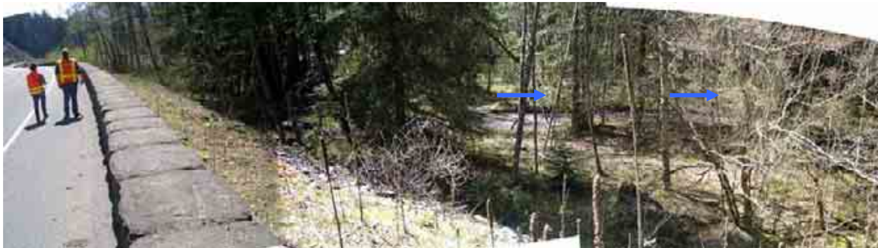
Site 2, MP 51.6. Side channel running along SR 410 embankment downstream of Skookum Falls Overlook. Areas of small deciduous trees such as right side of photo should be supplemented with large trees to prevent side channel from approaching highway embankment. April 25, 2005.
