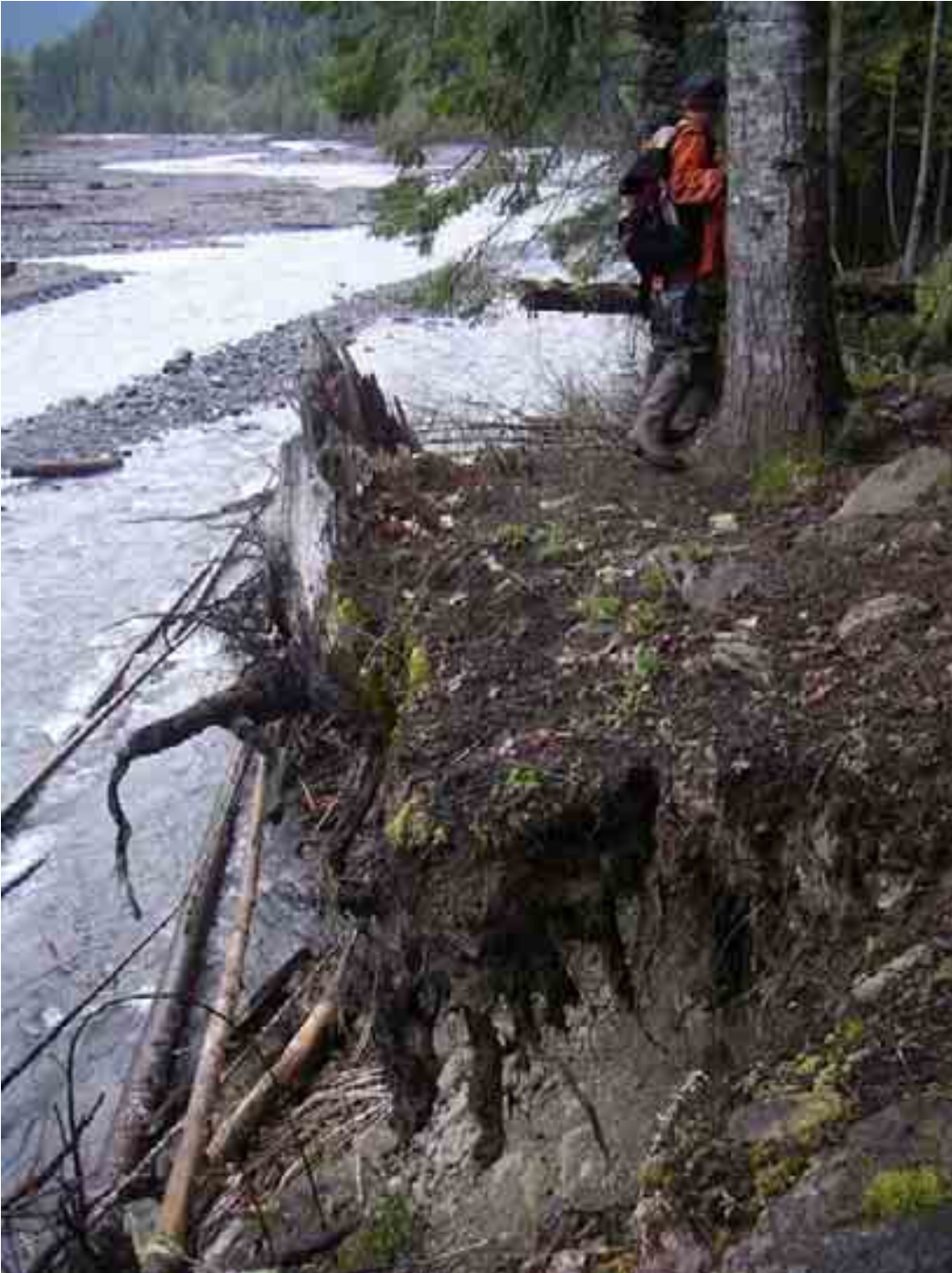
Site 7, MP 59.25. Looking downstream at severely undercut tree on eroding high bank along maintenance yard. April 27, 2005.
