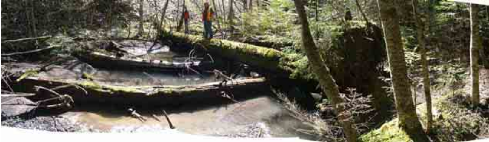
Site 2, MP 51.6. Example of natural LWD armoring at toe of SR 410 embankment, side channel downstream of Skookum Falls Overlook. April 25, 2005.
