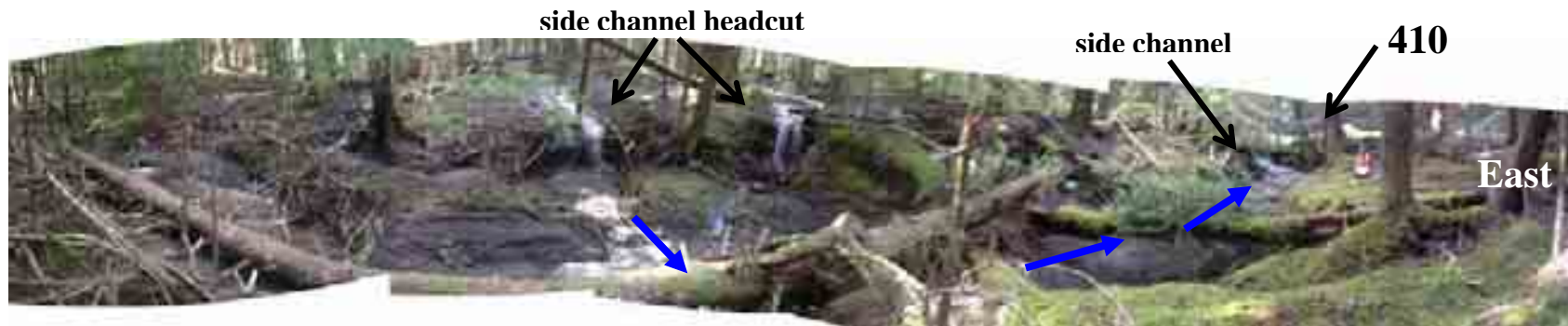
Site 4, MP 58.6 upstream headcut complex downstream of previous two photographs. Looking west from SR 410 near cross-section 7.
