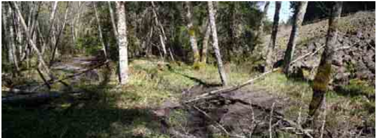
Site 2, MP 51.6. Side channel flowing along SR 410 embankment downstream of Skookum Falls Overlook. Inter-locking large trees should be placed at sites such as this where there are only sparsely spaced small trees to armor highway embankment and trap sediment. April 25, 2005.
