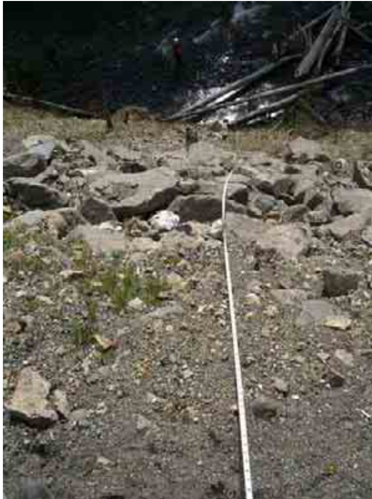
Site 3, MP 55 looking downslope approximately 90 feet from edge of pavement (EOP). Note lack of any woody vegetation on slope and edge of water at toe of slope. Most recent airphoto taken in 1998(?) shows approximately 100 feet of riparian forest between highway and river at this site. Rock riprap covers only upper 20 feet of slope and undercut by eroding slope. April 25, 2005.
