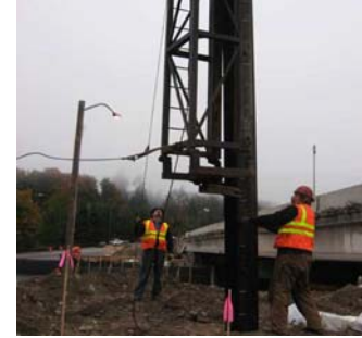
Crews drive piles near Coal Creek Parkway
