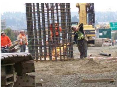
Crews build columns for the new southbound bridge over I-90
