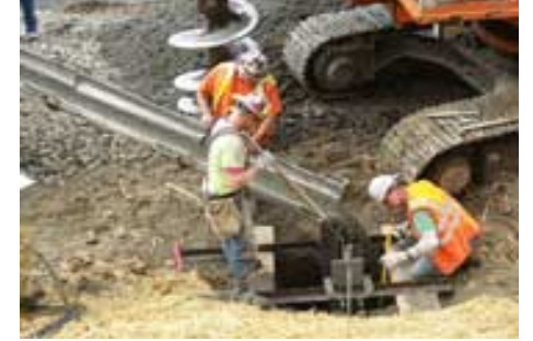
Crews pour concrete for a retaining wall near Coal Creek Parkway
