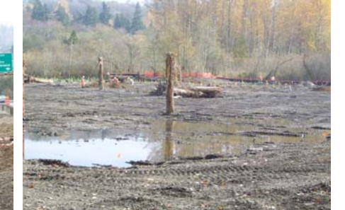
Crews amend soils at the Kelsey Creek wetland mitigation site
