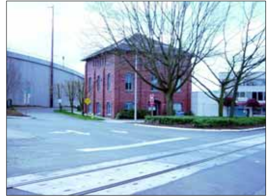
The Renton Substation of the Snoqualmie Falls Power Company
