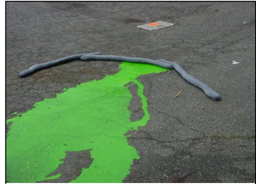
Socks prevent material from reaching storm drain
