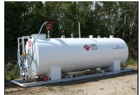
Double walled fuel tanks do not require secondary containment
