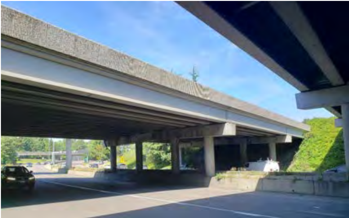
Bridge No 405/46W – I-405 over SR 520
