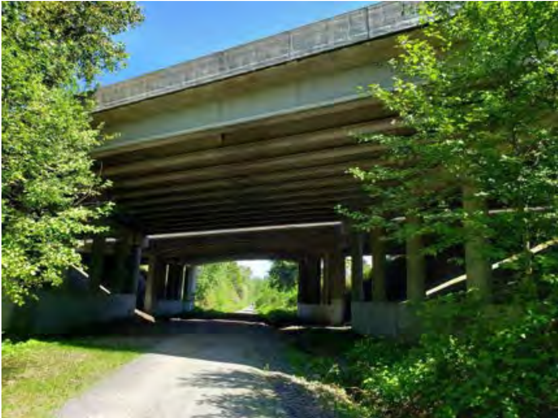
Bridge No 405/56W – I-405 over Pedestrian Trail
