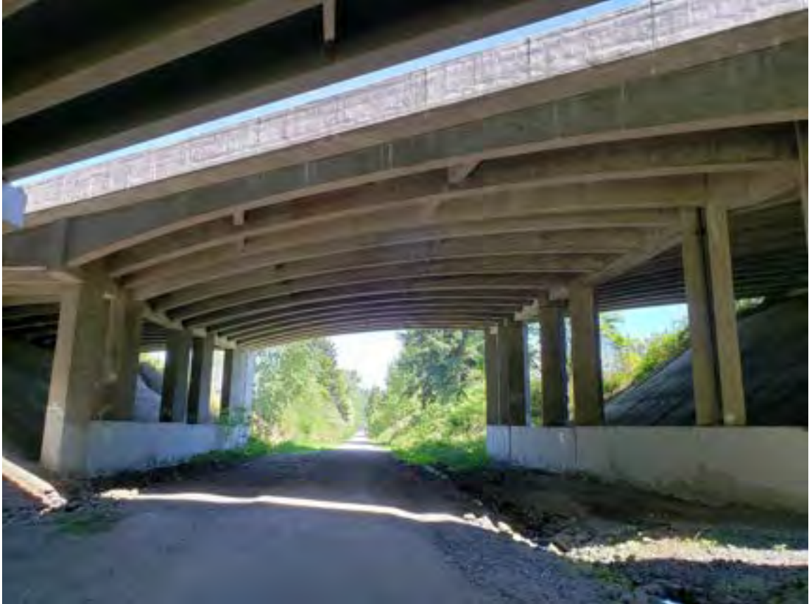
Bridge No 405/56E – I-405 over Pedestrian Trail
