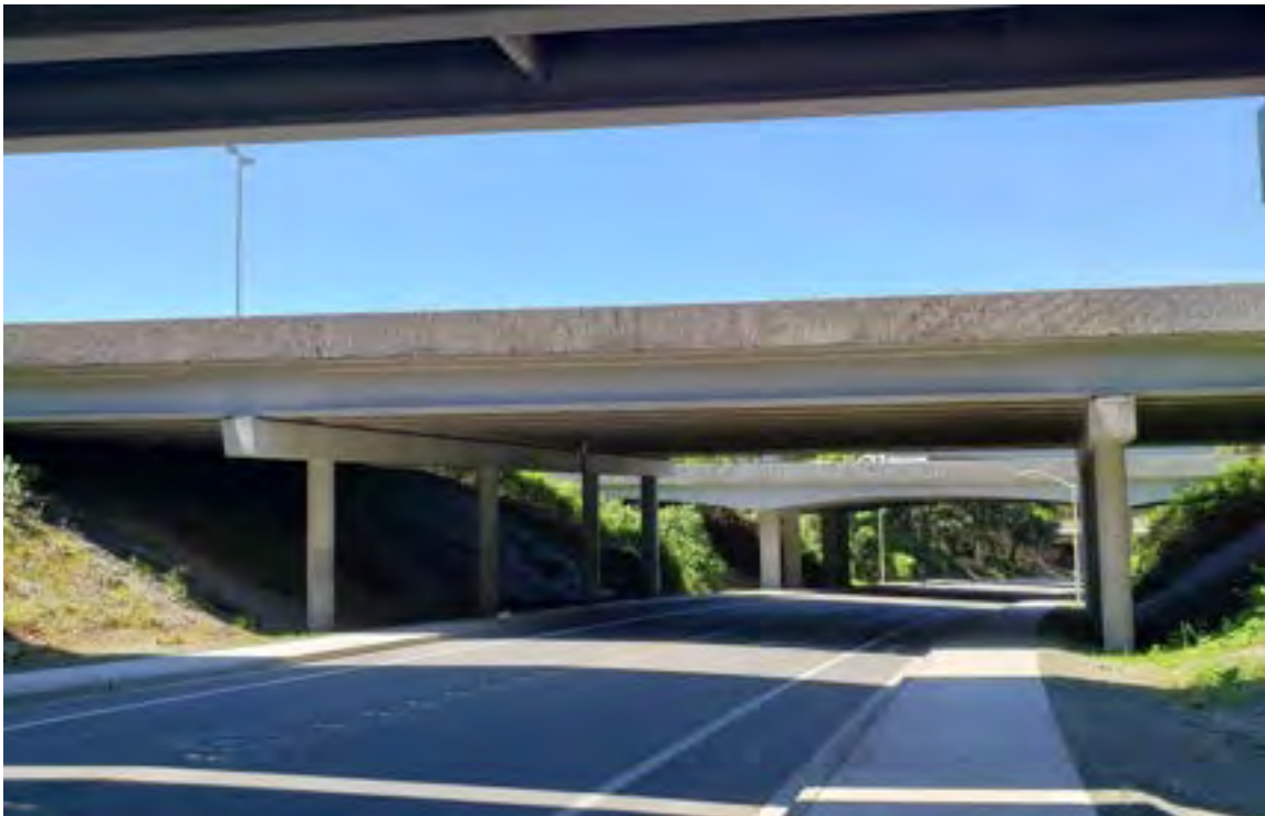
Bridge No 405/47E – I-405 over Northup Way
