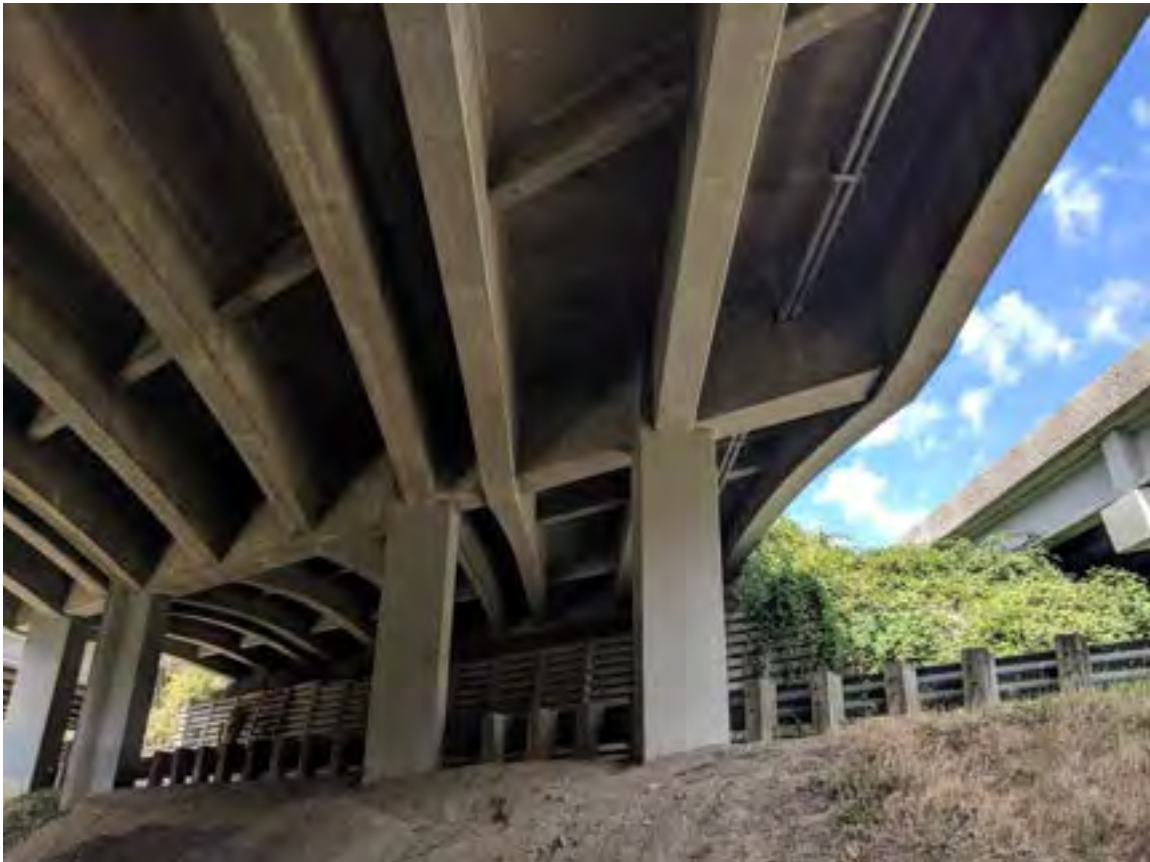
Bridge No 405/48W – I-405 over 115 th Ave NE
