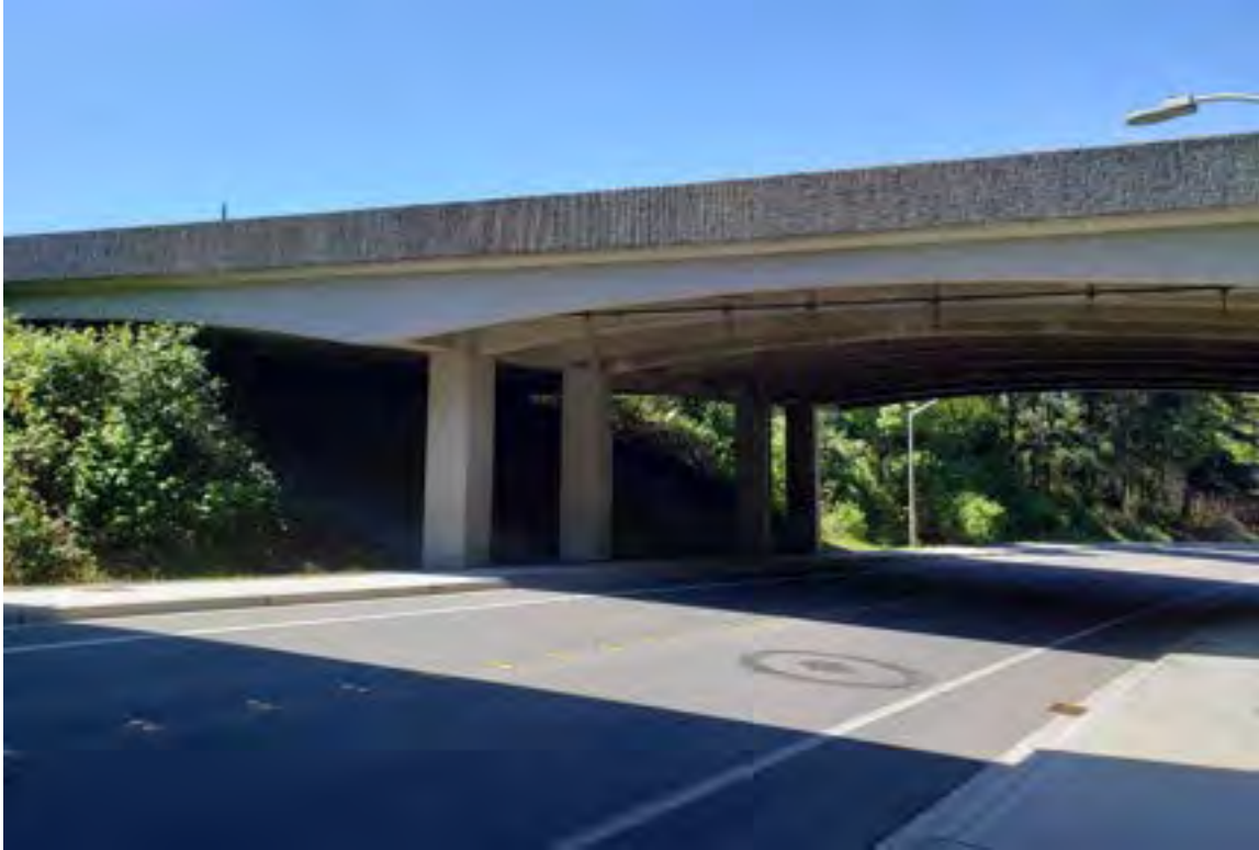
Bridge No 405/47W – I-405 over Northup Way
