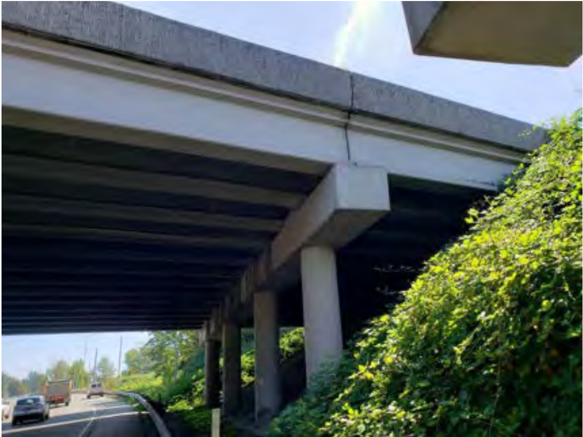
Bridge No 405/46E – I-405 over SR520
