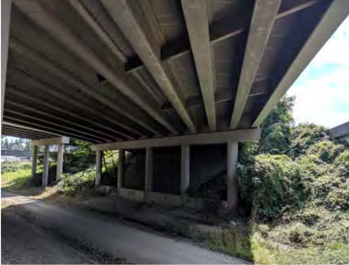
Bridge No 405/48E – I-405 over 115 th Ave NE
