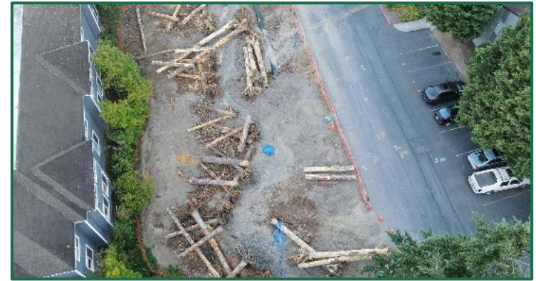
Wood placement is a critical step in the fish barrier correction process
