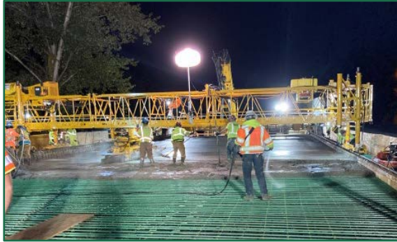
Northeast 44 th Street Interchange
