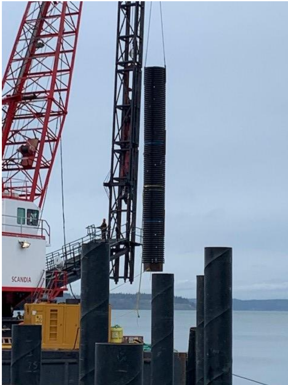
Figure 5: Confined Bubble Curtain Used at Mukilteo Ferry Terminal Project
