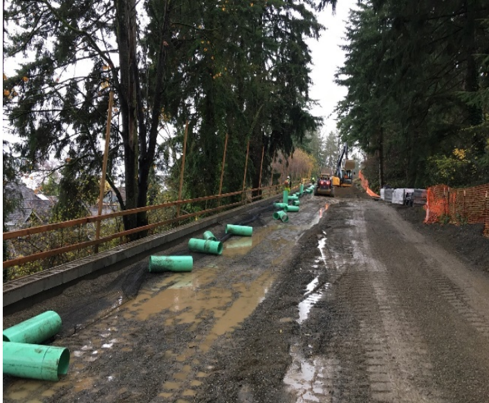
King County Eastrail progress: construction & grading
