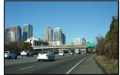
Existing Main Street Overpass
