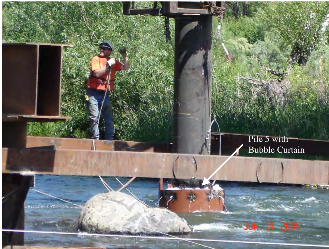
Figure 10: Pile 5 with Bubble Curtain in Operation.
