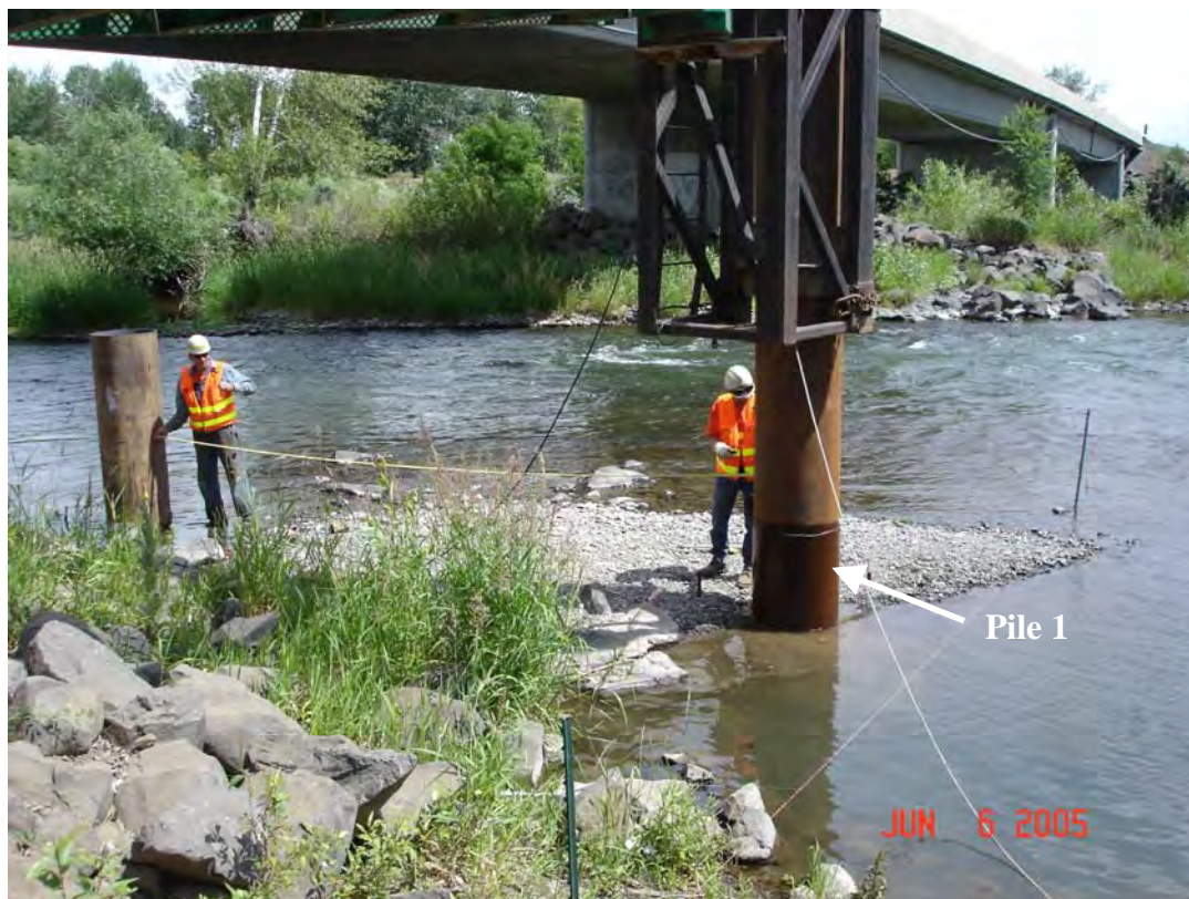
Figure 6: Location of Pile 1 at waters edge.
