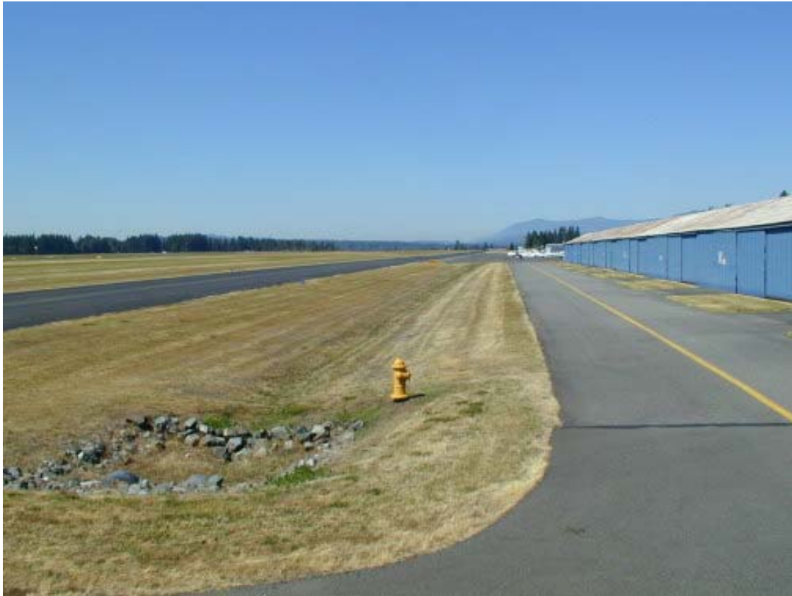
Vegetated filter strip in along airport runway.
