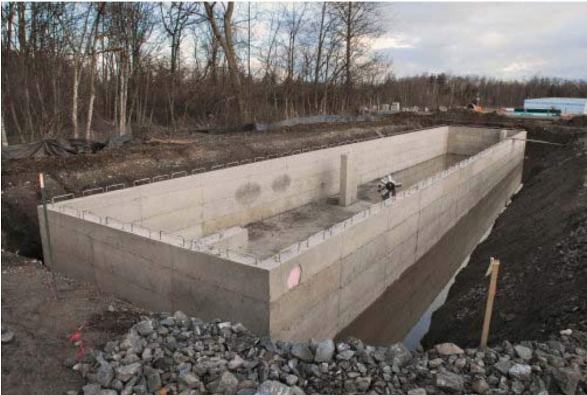
Detention vault during construction at Bellingham.
