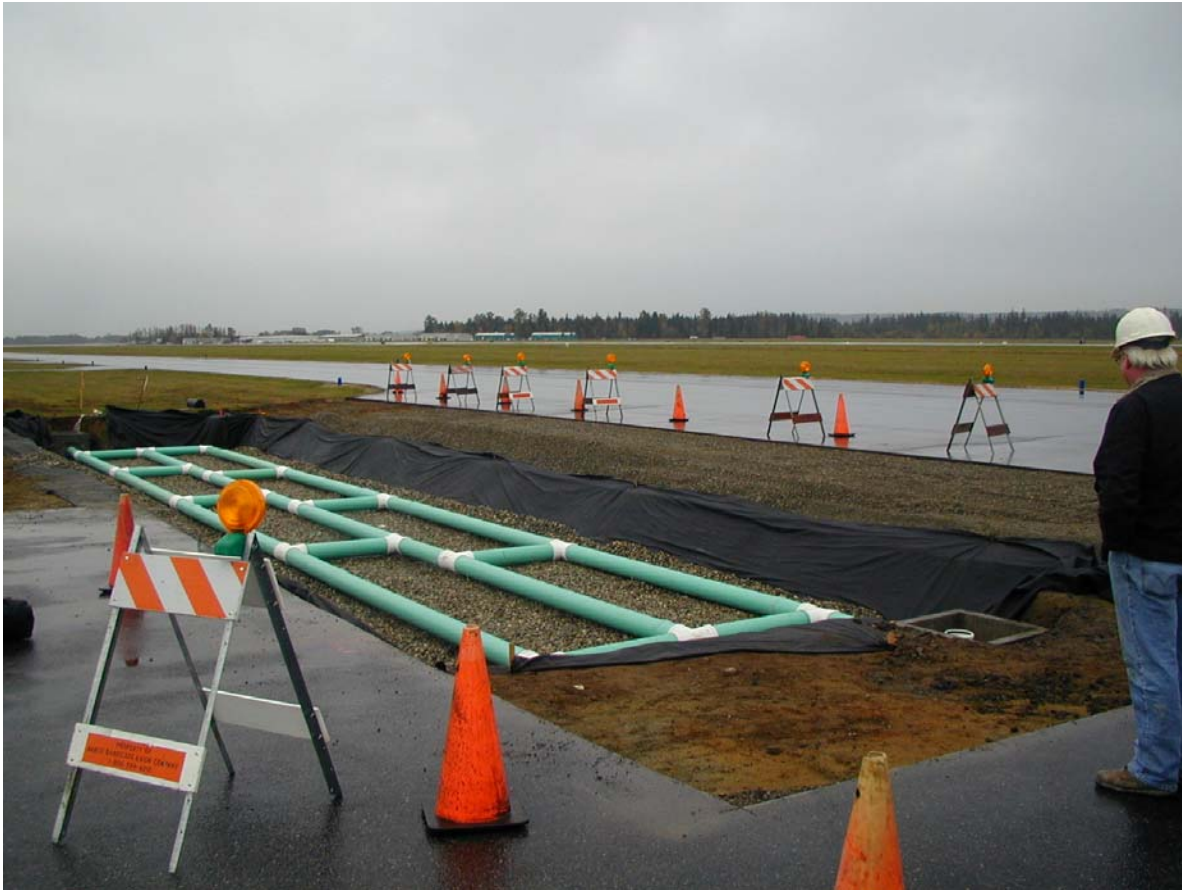
Underground infiltration installation at Arlington airport.
