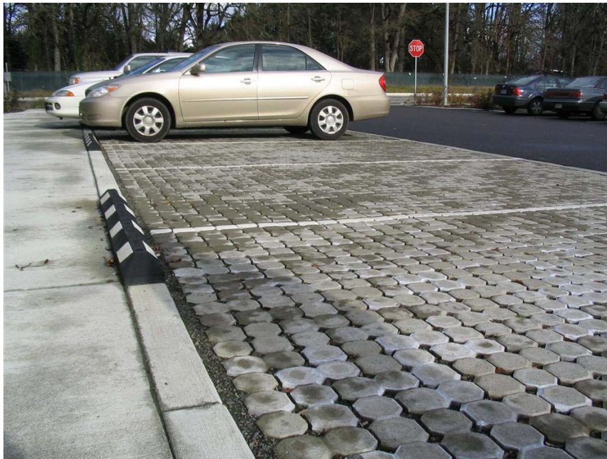
Use of porous pavers in parking lot.
