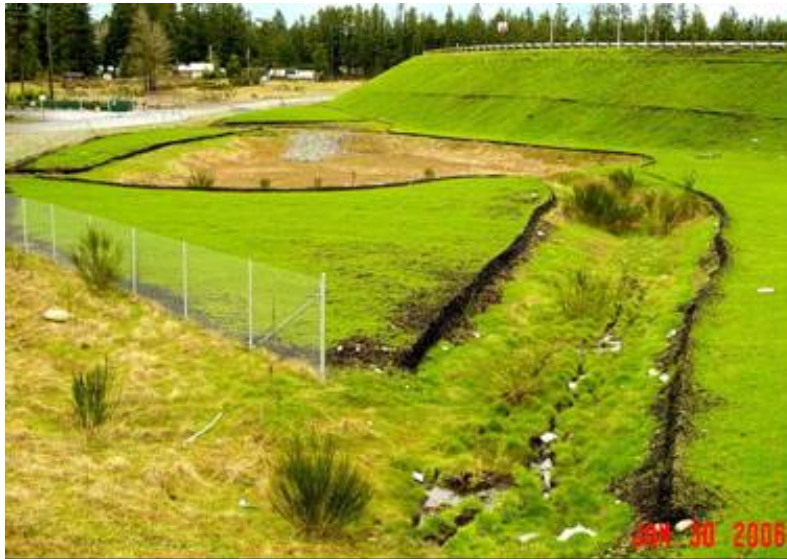
Bioinfiltration pond with Bioswale.
