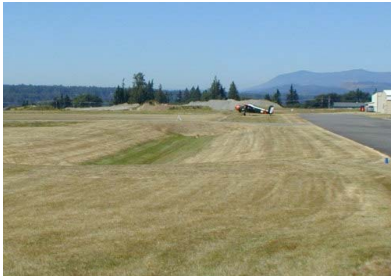
Biofiltration swale along taxiway.
