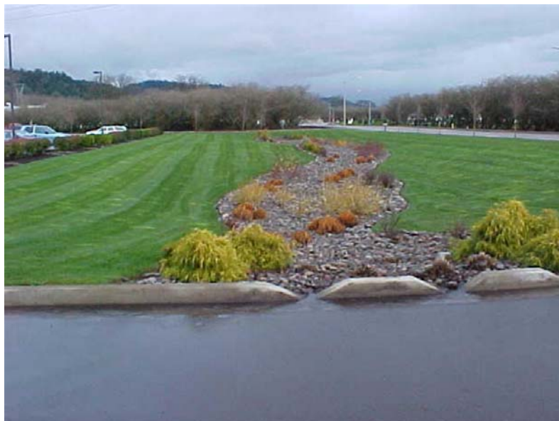
Biofiltration swale at industrial facility.
