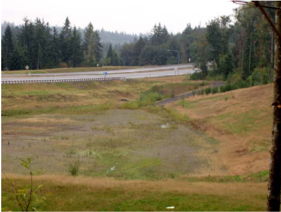
Detention pond Along SR 18 in King County.
