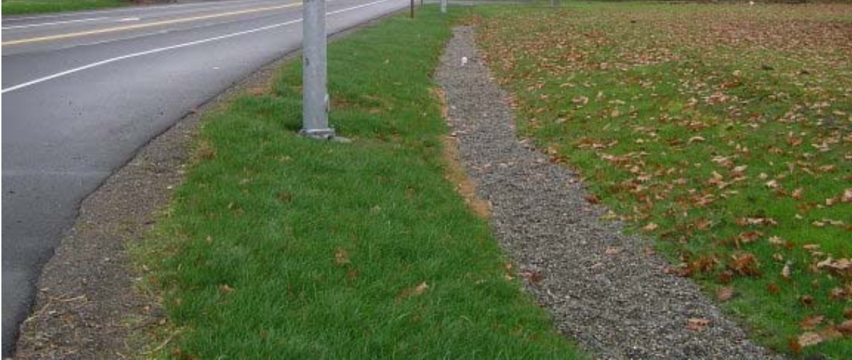
Infiltration trench along SR 539.
