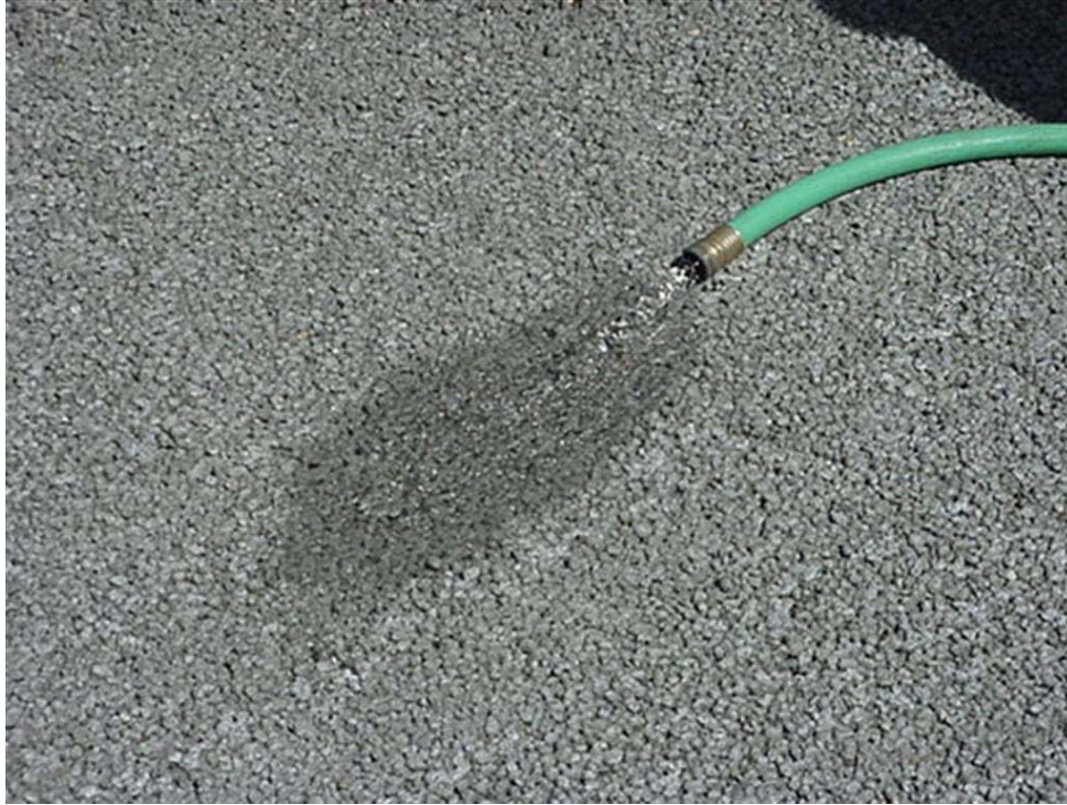
Porous concrete showing rapid infiltration.
