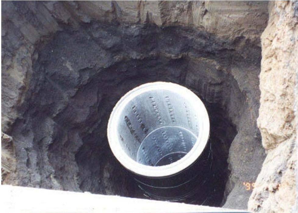
Drywell installation.
