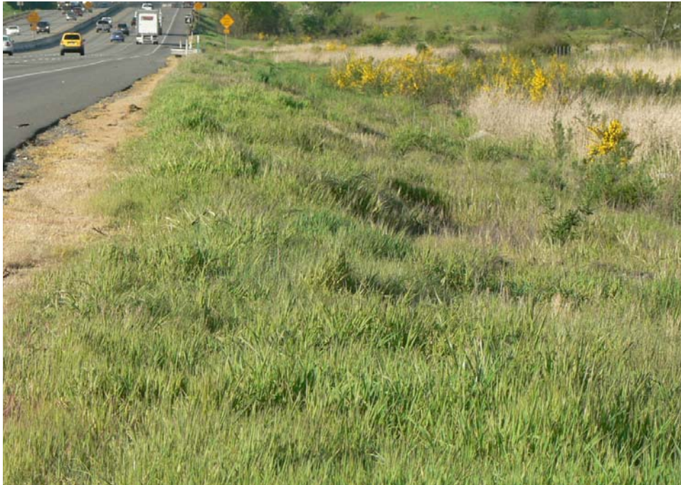
Engineered Dispersion Area Along I-5.
