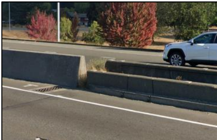
Photo A: Need for Mitigation - Single Slope Barrier Adjacent to Shorter Bridge Barrier
