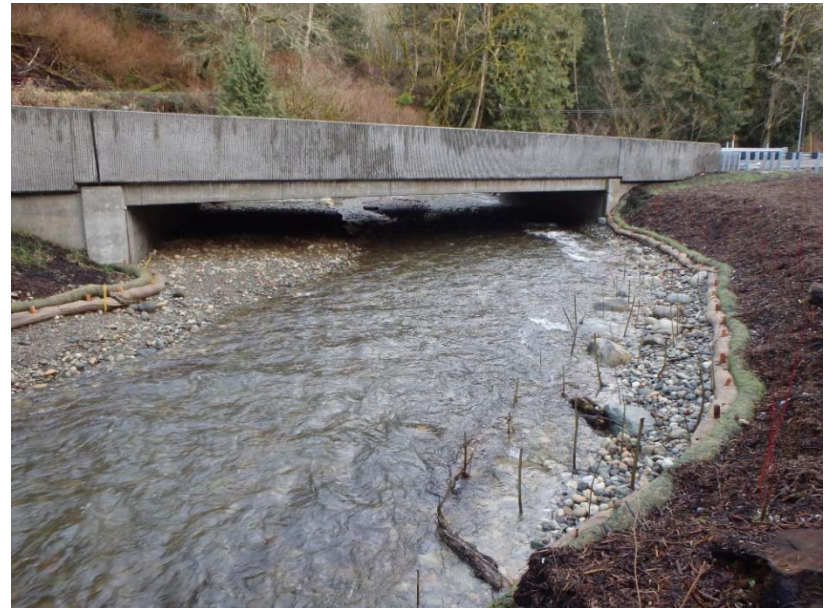
Top: SR 542 High Creek, built 2016 Bottom: SR 9 Lake Creek, built 2015
