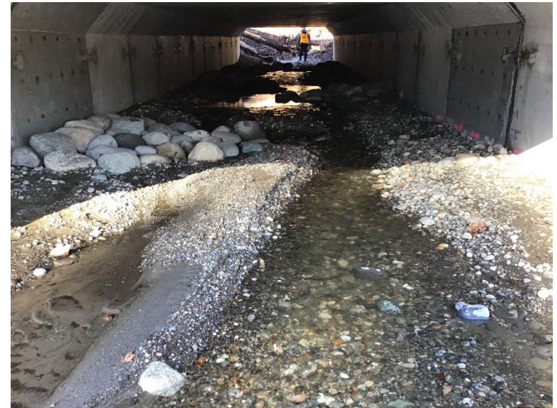
SR 9 Norway Park Creek, Built 2022
