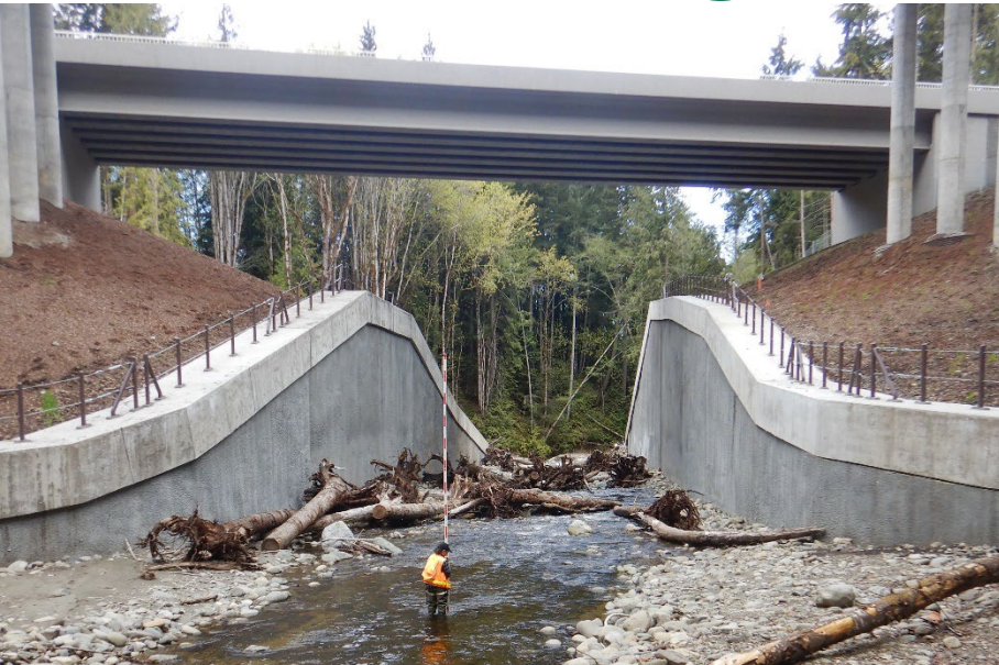
US 101 Siebert Creek, built 2020-2021
