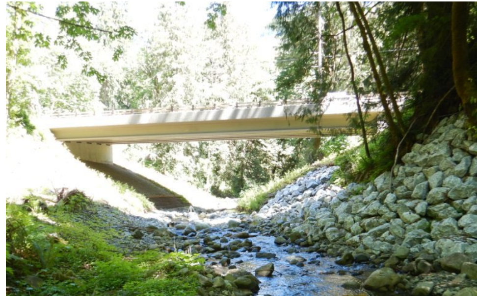
SR 542 Hedrick Creek, built 2018
