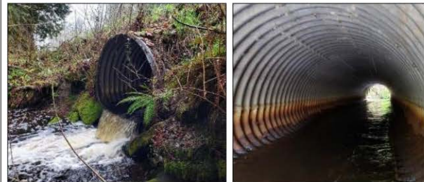
Figure 9 Culvert outlet (left), inside view of culvert (right)
