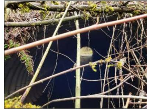
Figure 8 Culvert inlet looking downstream
