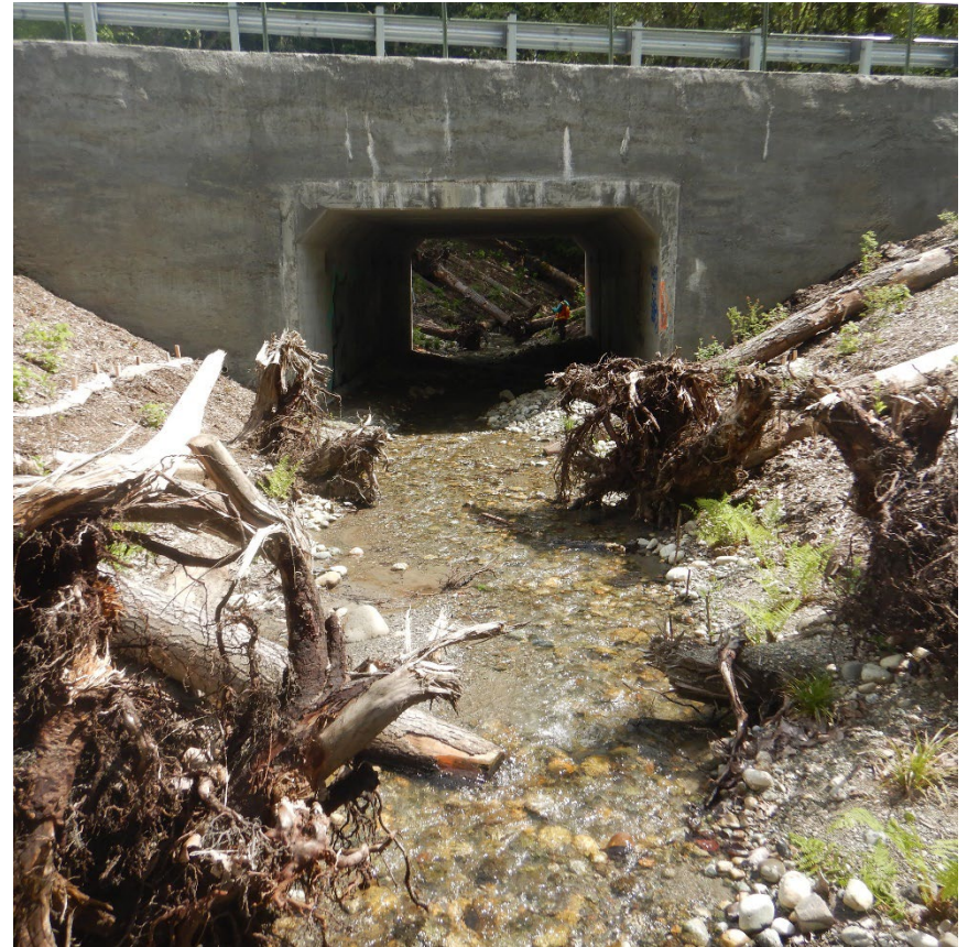
SR 20 Lorezan Creek, Built 2021
