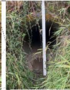
Existing 48-inch outlet
