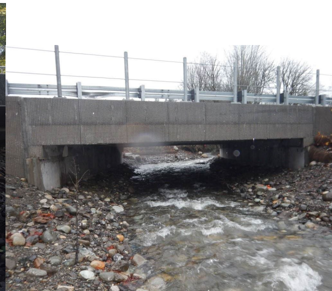
SR 542 High Creek, Built 2016
