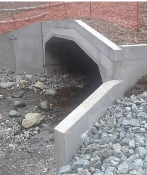
SR 532 Church Creek, Built 2017
