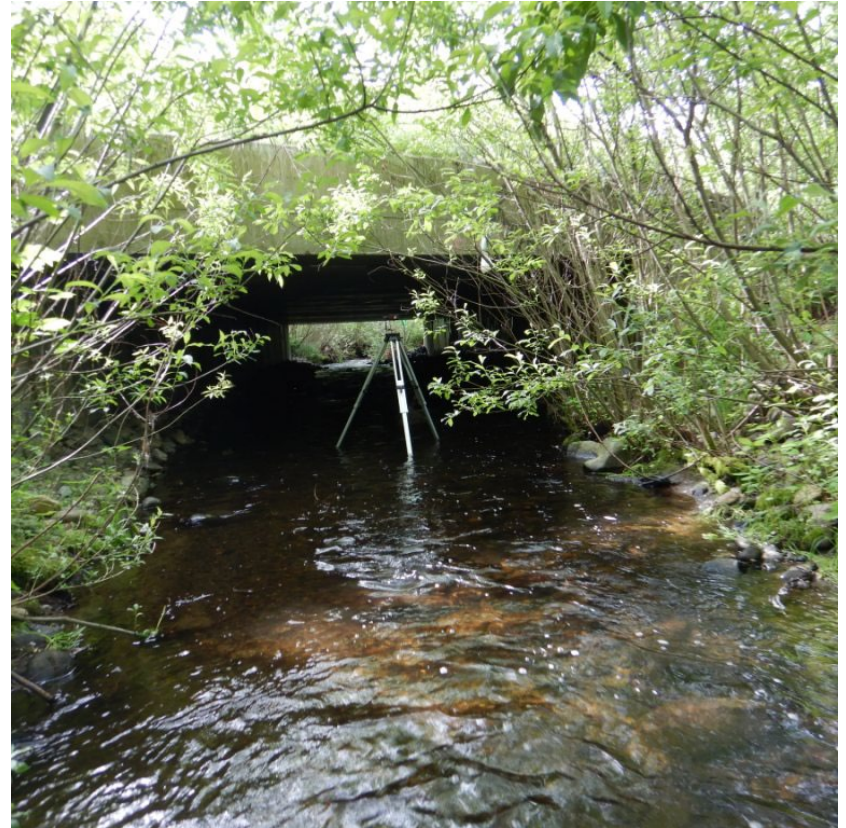
SR 99 WF Hylebos Creek, Built 2015
