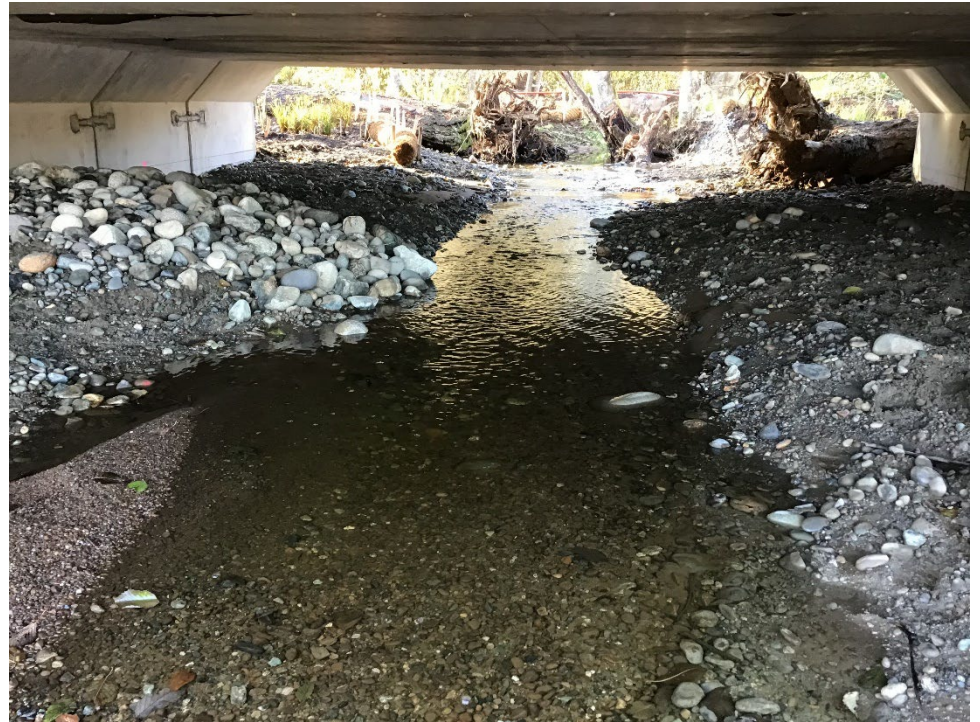
SR 9 Lake Creek, Built 2022
