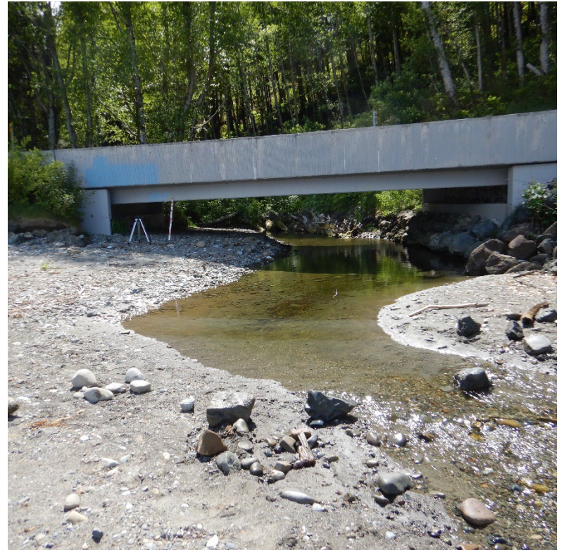
SR 112 Jansen Creek, Built 2016
