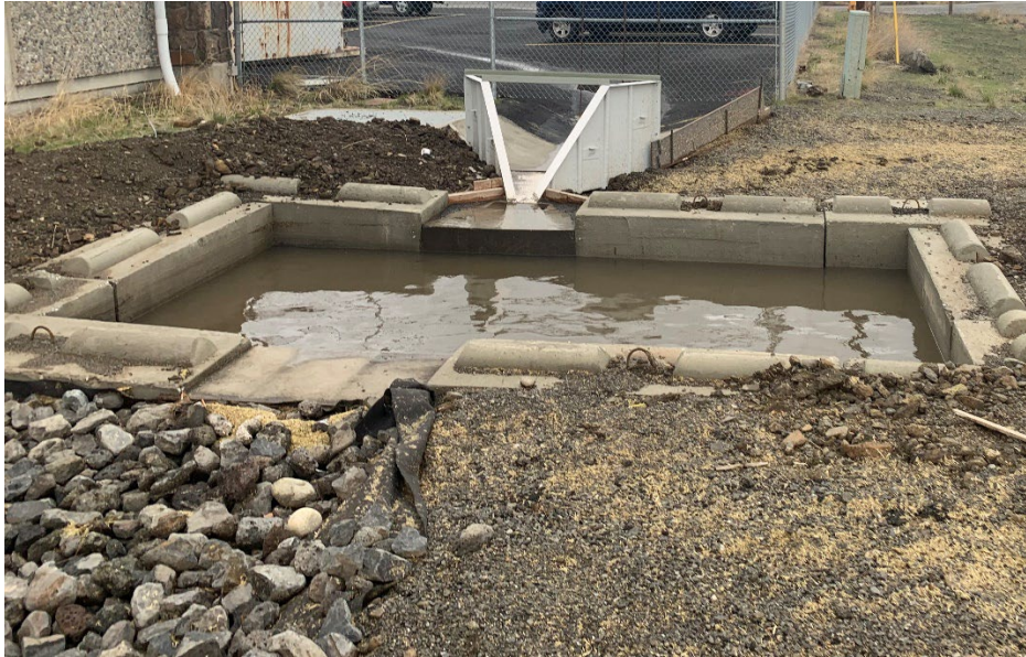
Figure 5. Geiger influent with siltation basin
