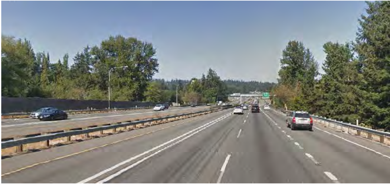
Exhibit 4-8. Northbound I-405 Approaching SR 527
