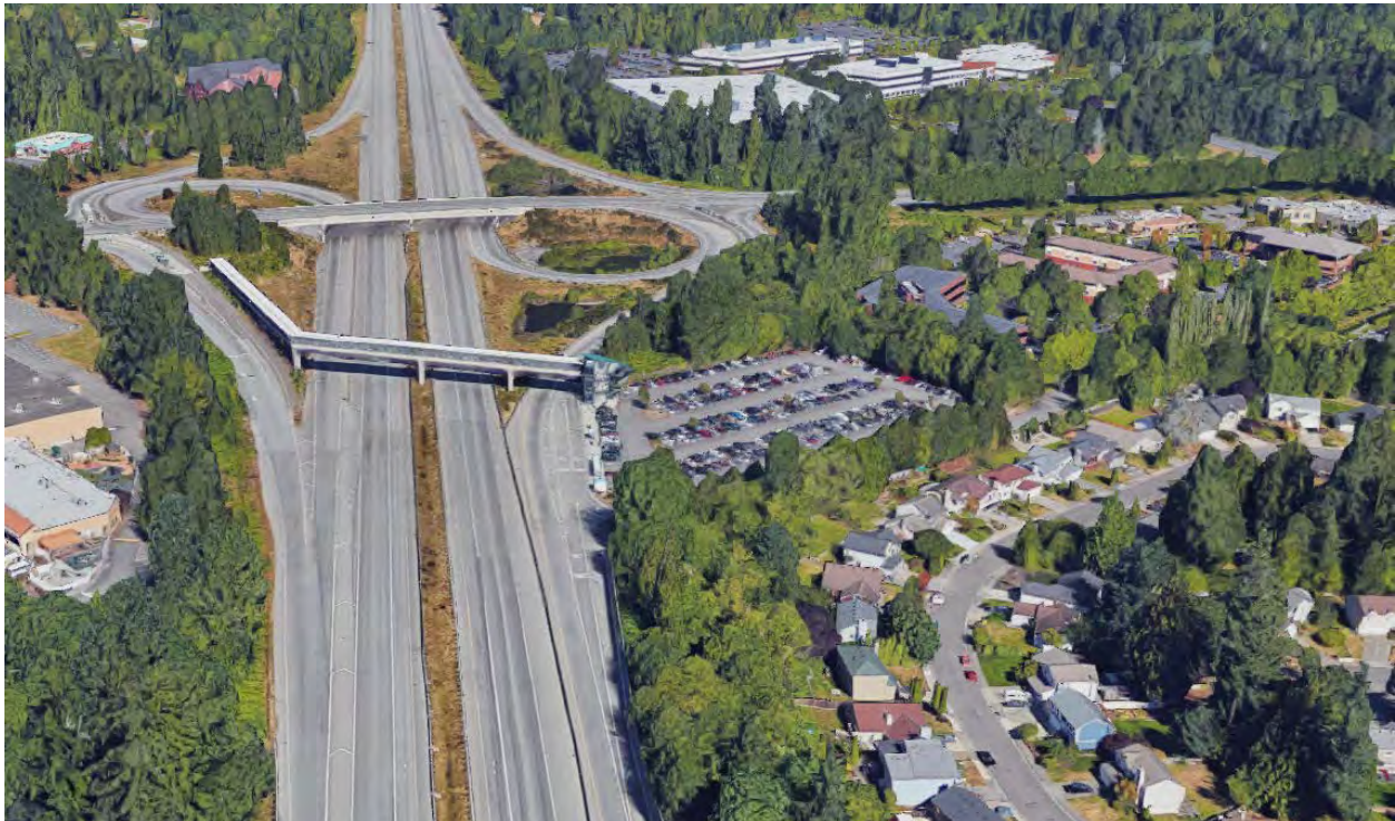
Exhibit 5-9. Aerial View of Existing Conditions near I-405/SR 527 Interchange
