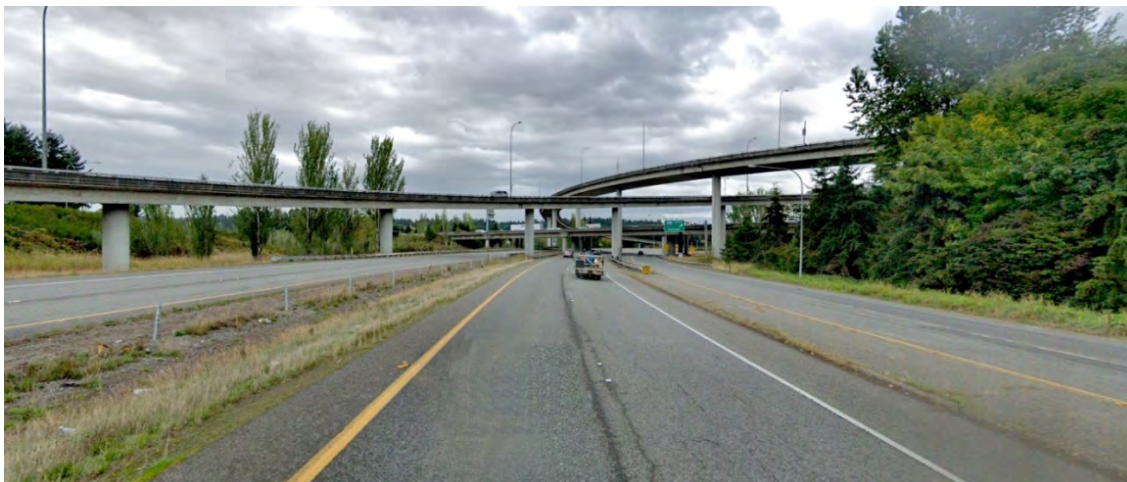
Exhibit 5-7. Existing Conditions Approaching I-405/SR 522 Interchange Viewed from Eastbound SR 522
