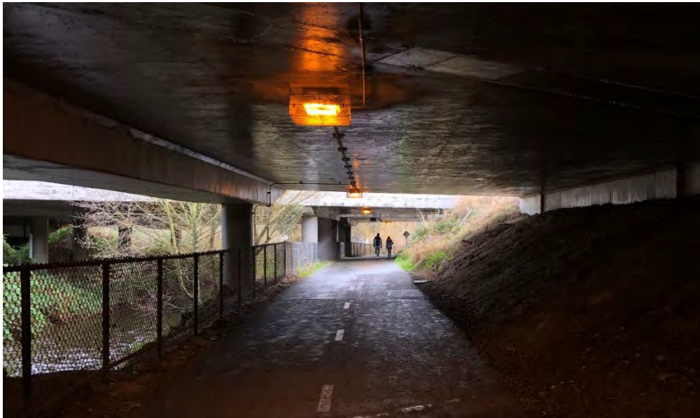
Exhibit 5-5. Existing Conditions North Creek Trail Underpass at SR 522
