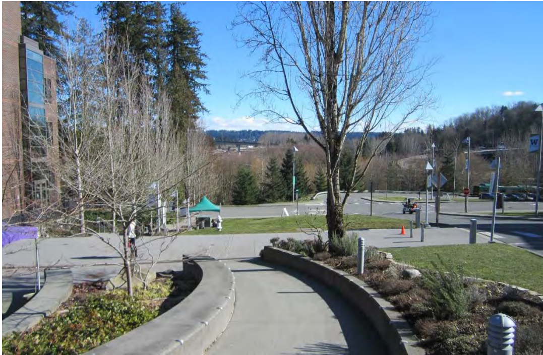
Exhibit 4-5. I-405/SR522 interchange Viewed from UW Bothell Campus Path
