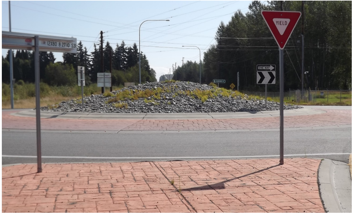
Roundabout with hardscape- reduces life cycle/maintenance costs.
